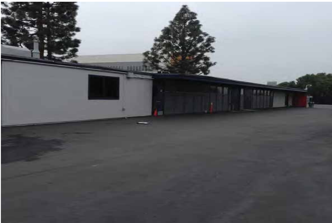
Photograph 5-General view of the suspect roof and exterior building materials, building 110
