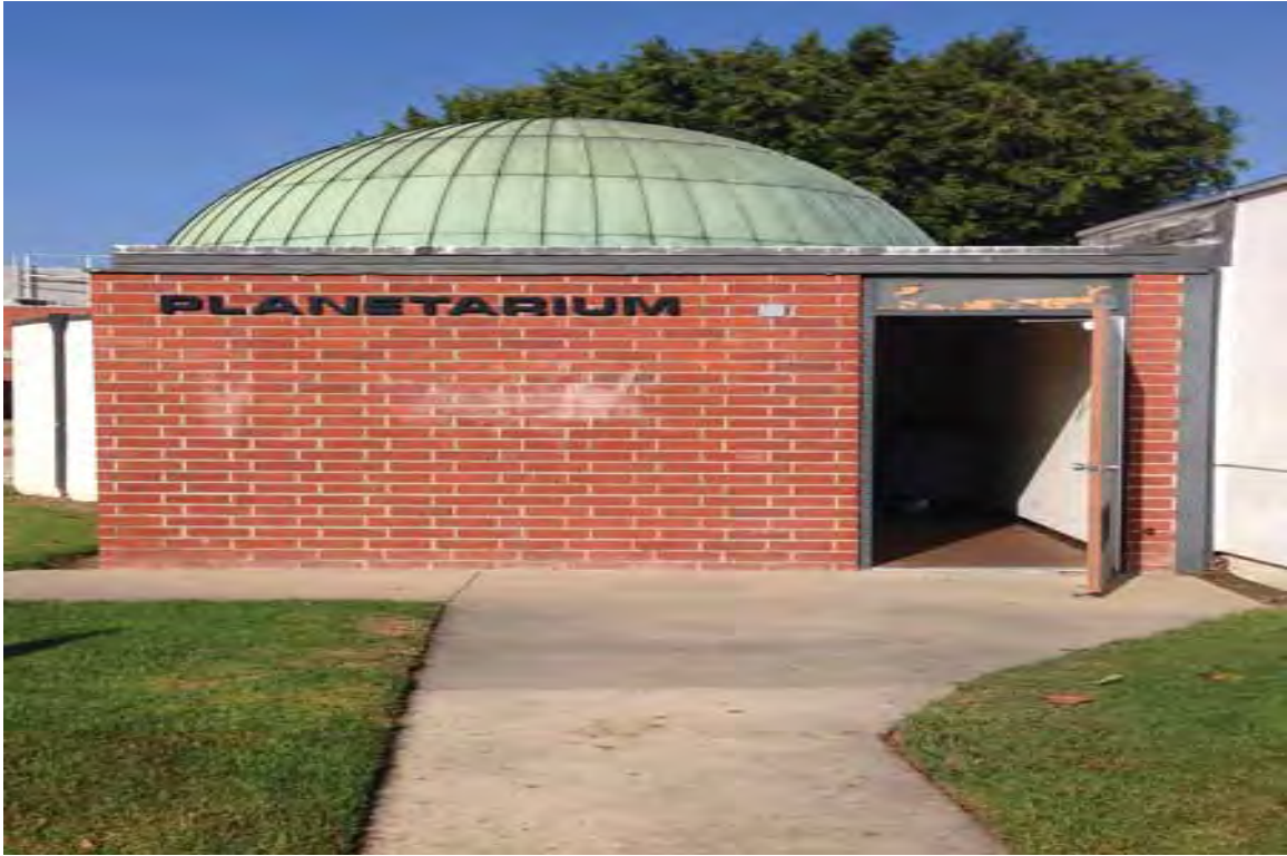
Photograph 12-General front view of the building 39
