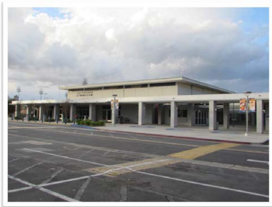
PHOTO - 26: Gymnasium complex, looking northwest, 2014.
