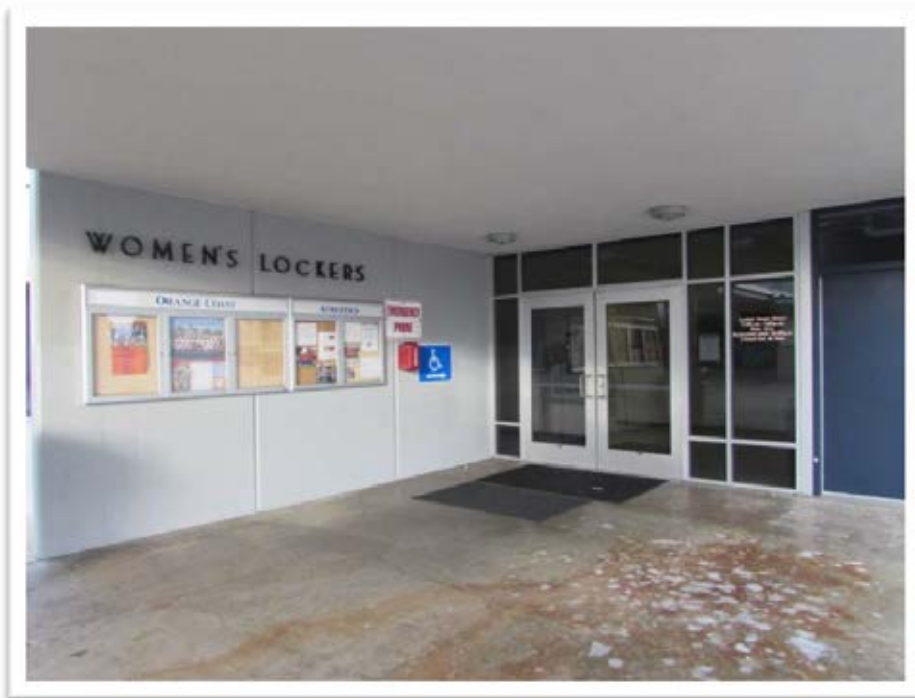
PHOTO - 28: Women's Locker Room entry, looking northeast, 2014.
