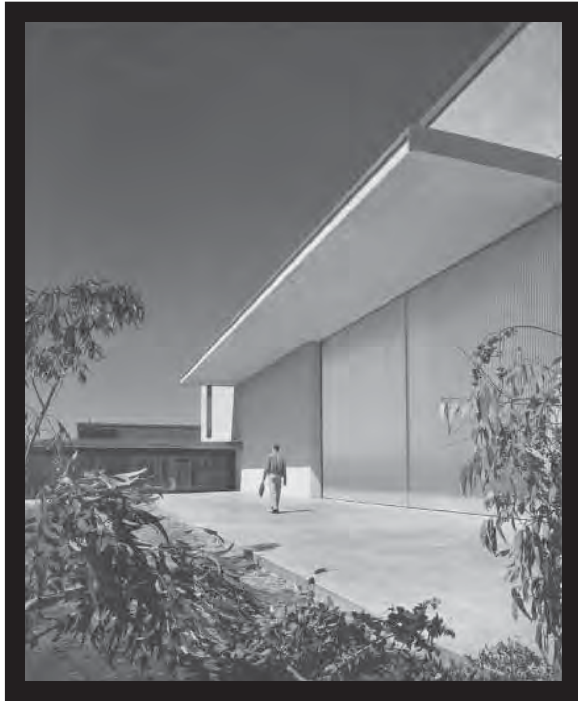
South elevation of the Theater (Robert Moore Theater, Bldg. 2); ca. 1955. Julius Shulman Photography Archive. Copyright The J. Paul Getty Trust. The Getty Research Institute, Los Angeles.
