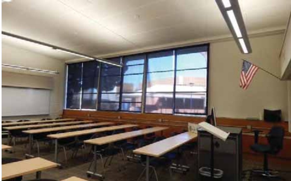
Figure 1C-37: Typical classroom in Building 12 and 13. Note the shear wall at the right.
