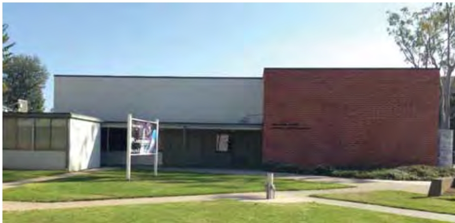
Figure 1C-79: West façade of Building 37 with Building 38 at the left.
