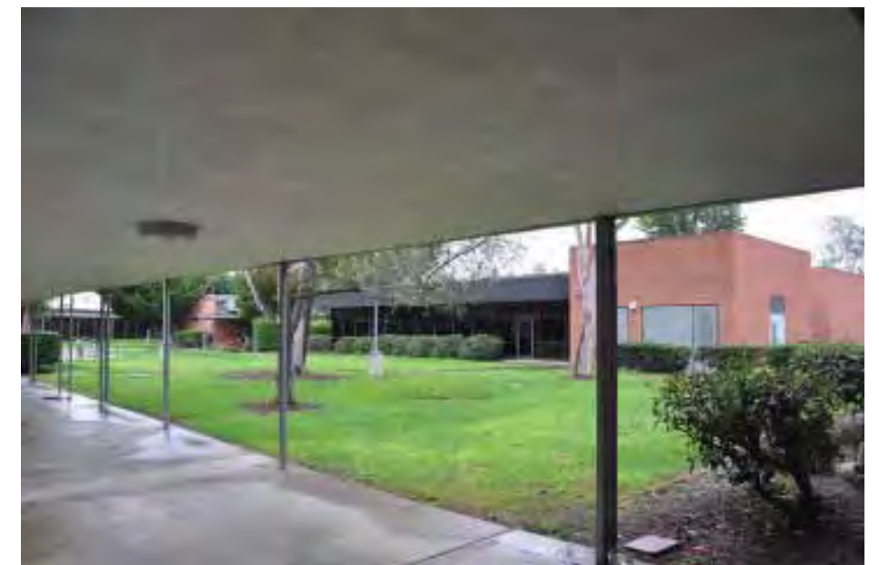
Figure 20: View of Building 14 addition from covered walkway, 2015. Source: Page & Turnbull.
