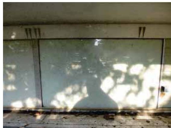
Figure 173: Blocked clerestory window on Building 36.
