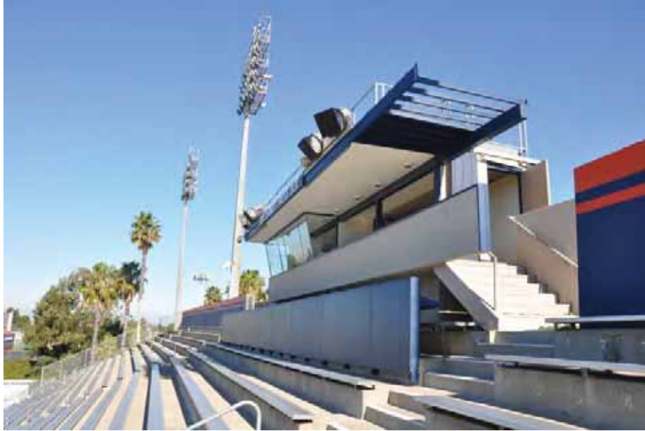
Figure 1C-106: East press box with canted glass, extended trellis, and Flexboard fascia, looking north.
