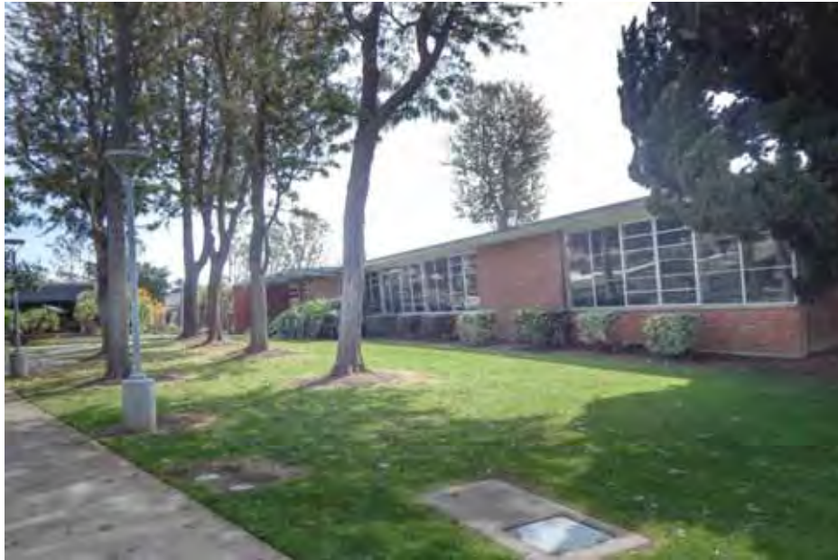
Figure 1C-34: North façade of Buildings 12 and 13, looking southeast. Showing angled aluminum framed windows and brick walls with slightly corbeled sections.
