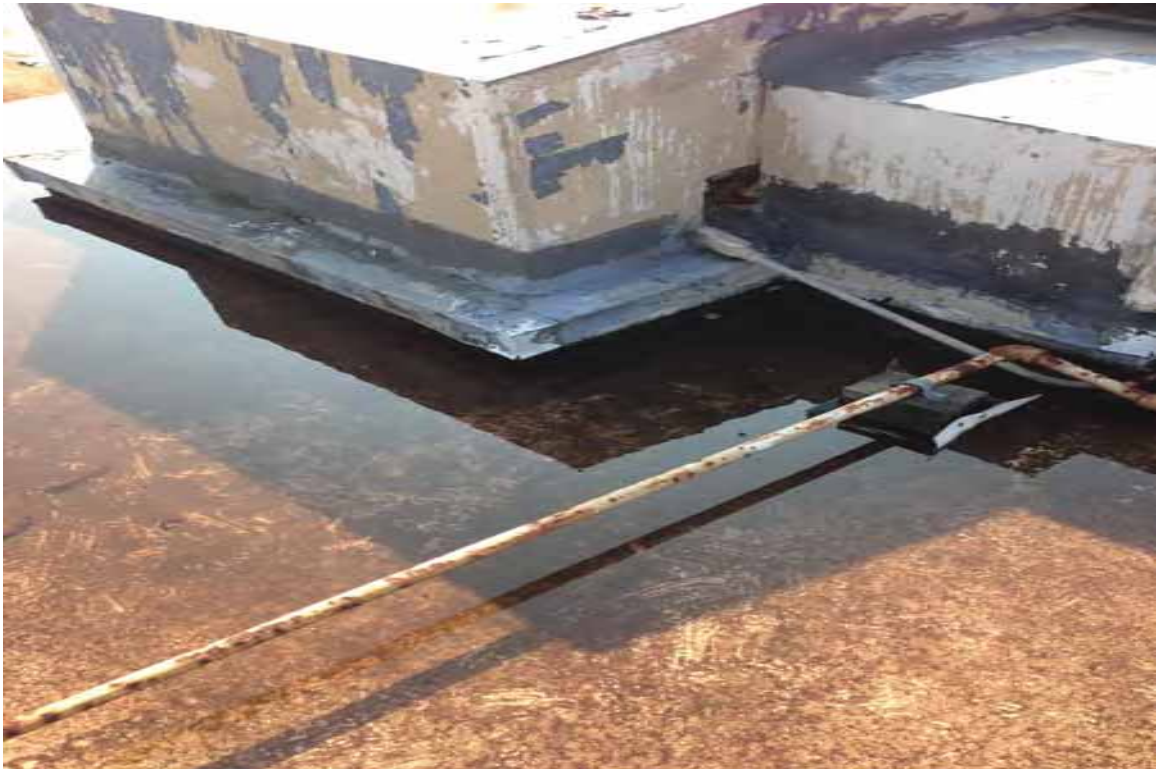
Photographs 16-General view of the suspect roofing materials
