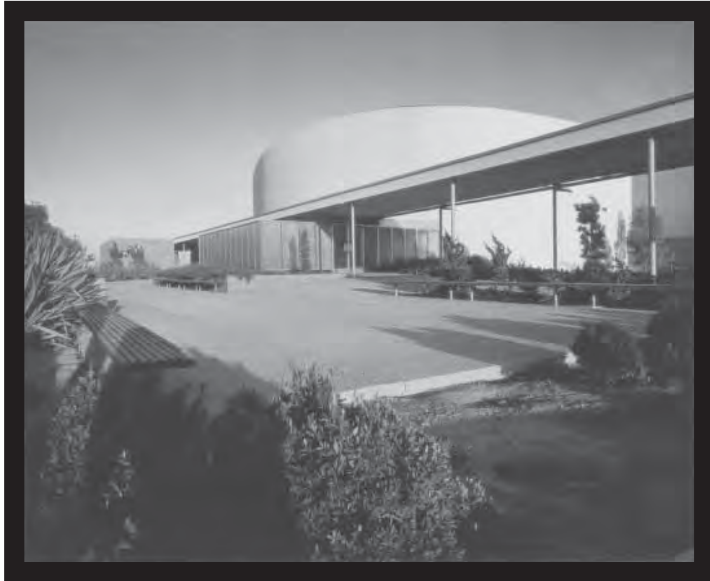
North elevation of the Theater (Robert Moore Theater, Bldg. 2); ca. 1955. Julius Shulman Photography Archive. Copyright The J. Paul Getty Trust. The Getty Research Institute, Los Angeles.
