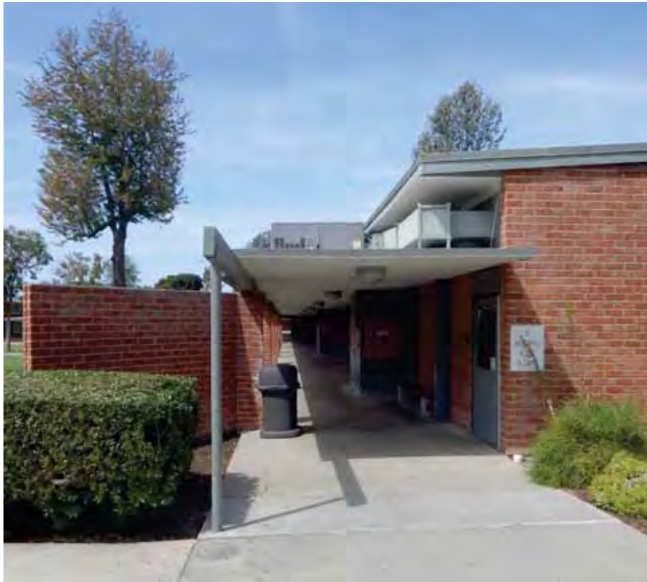
Figure 1C-33: South façade of Buildings 12 below covered walkway supported by brick wing walls. HVAC ducts are in the clerestory windows above the covered walkway.
