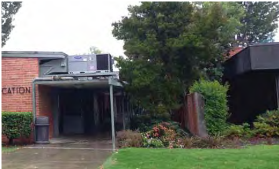
Figure 1C-41: Brick screen wall between Building 13 (left) and Building 14 (right) with planting strip, looking east.
