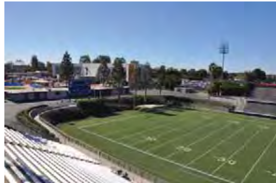
Figure 1C-105: South end of the Stadium showing grade transition and vehicle ramp, looking southeast.
