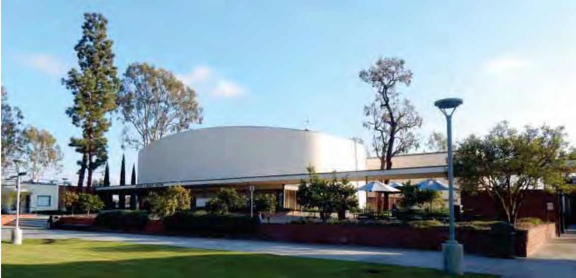
Figure 145: North façade of Robert Moore Theater (Bldg. 2), center, and west façade of Ticket office (Bldg. 2b), left.
