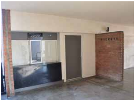
Figure 1C-55: Ticket window and perpendicular brick wall at Building 2B's south façade.
