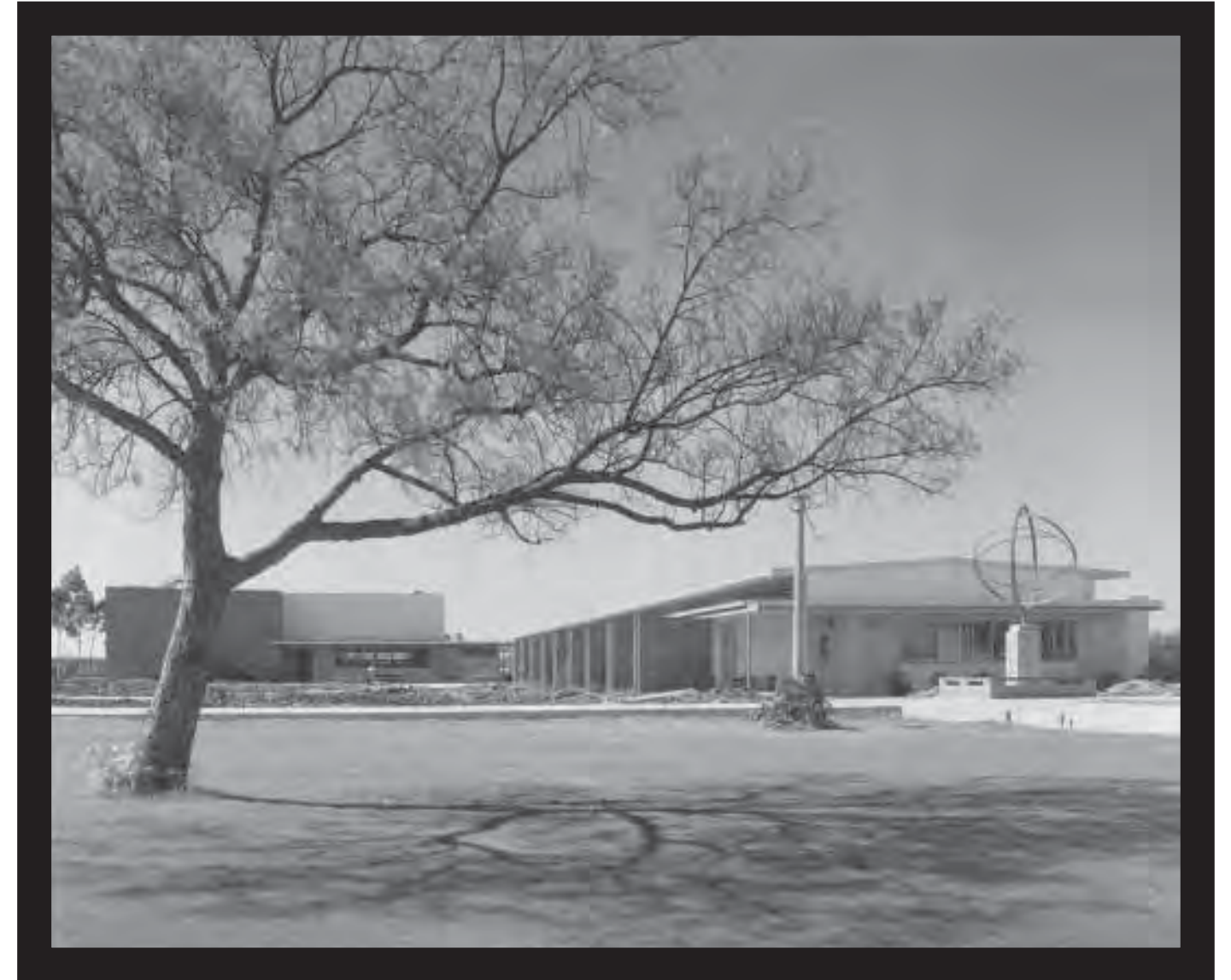
South elevation of the Science Building (Math Wing and Reprographics, Bldgs. 35 and 37); ca. 1957. Julius Shulman Photography Archive. Copyright The J. Paul Getty Trust. The Getty Research Institute, Los Angeles.
