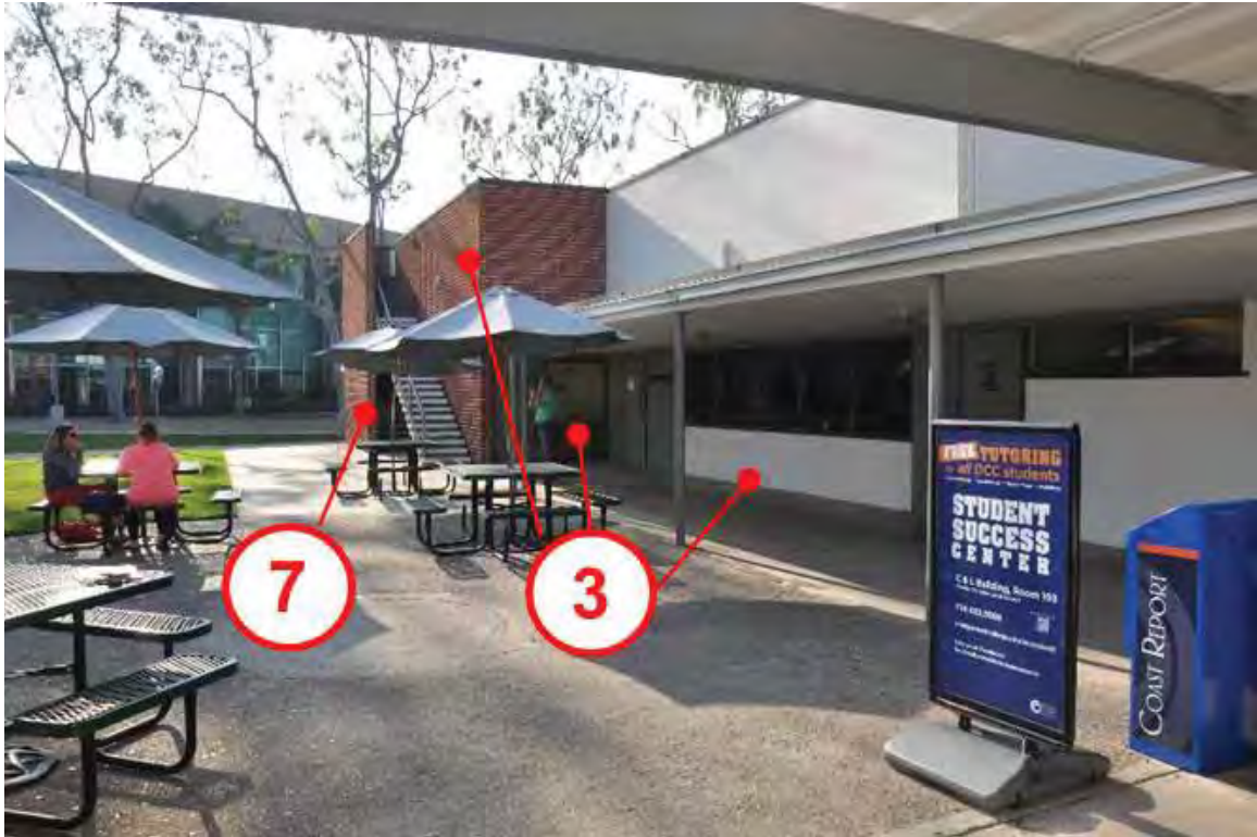
Figure 1D-24: Contemporary image of the Reprographics Building (Bldg. 37) with character defining features identified by red callouts.
