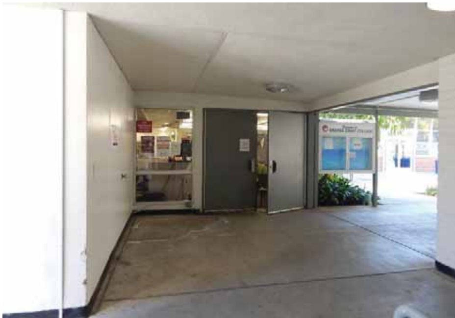
Figure 1C-11: Vestibule to Building 7's main entrance at the north elbow of the building, looking plan south. The right openings leads to Building 7's courtyard and Building 8's south covered walkway.
