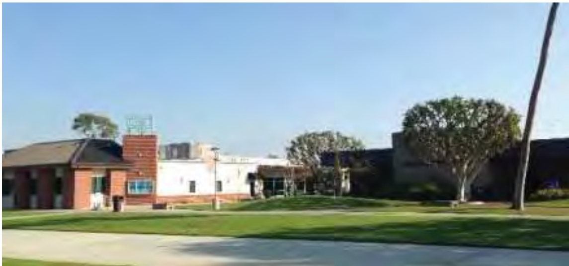
Figure 1C-117: The altered Student Center (Bldg. 86, 1953, altered ca. 1992) and Administration (Bldg. 1, ca.1975) east of the Historic District, looking north.
