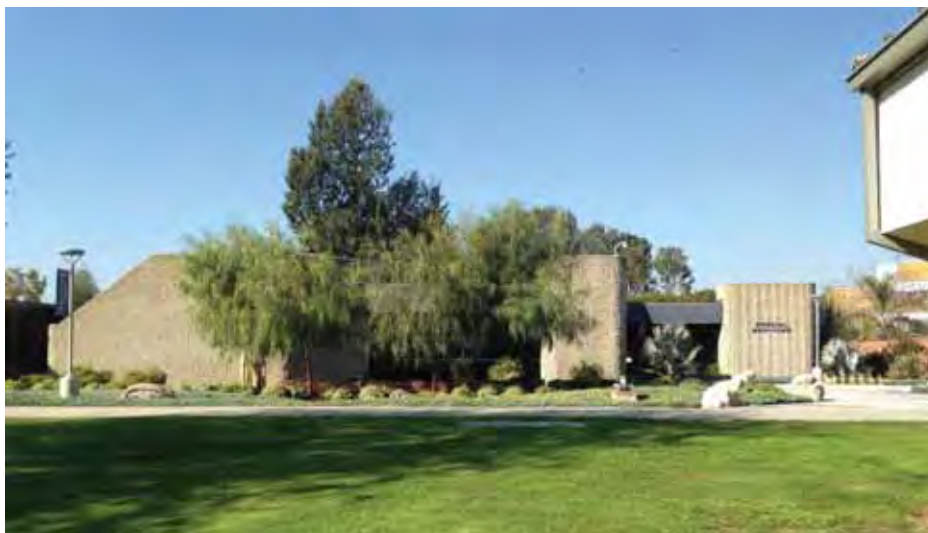
Figure 1C-112: The Student Service Center constructed after the period of significance.
