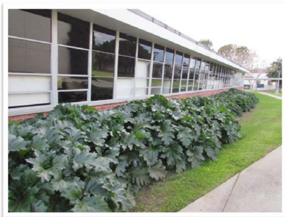
PHOTO - 36: Classroom window and planting details, 2014.
