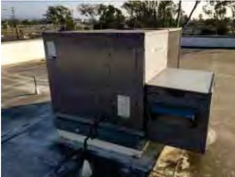
Typical DX Rooftop Packaged Unit
