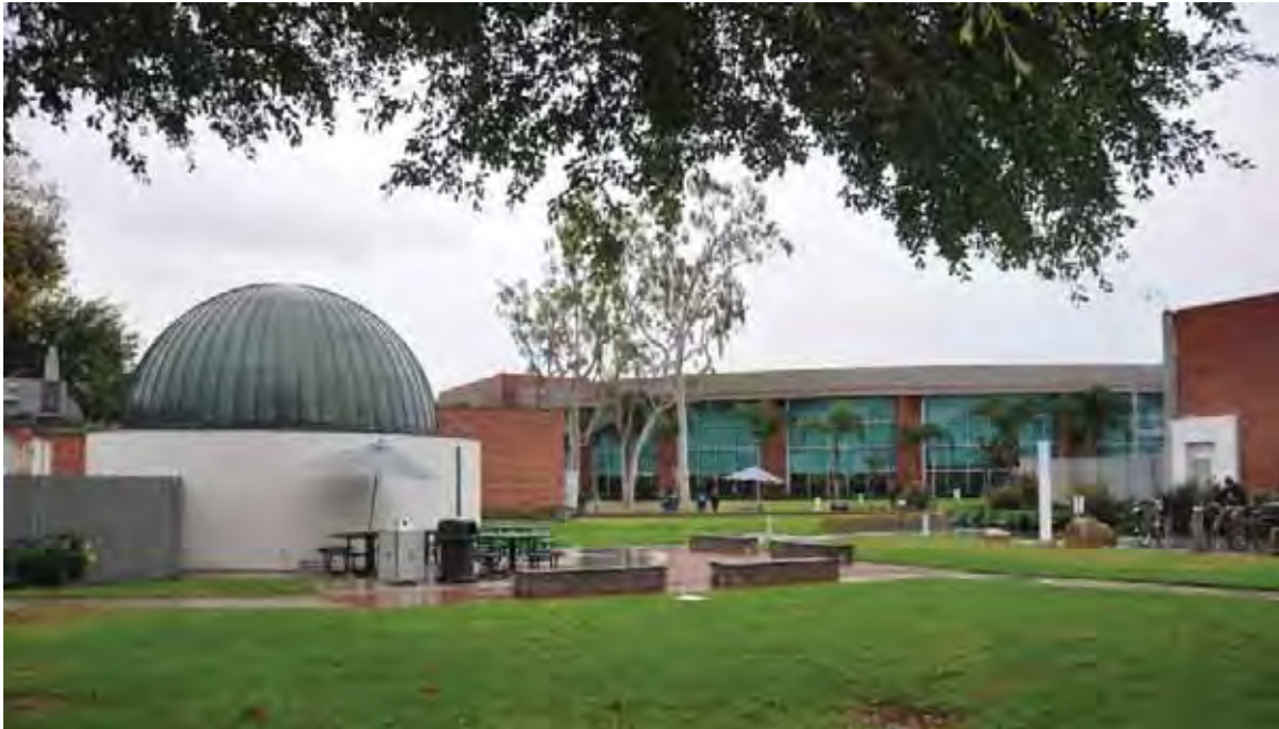
Figure 1C-118: Library (Bldg. 182, 2008) south of the Historic District, looking southeast. The Historic District's Planetarium (Bldg. 39) is in the foreground.
