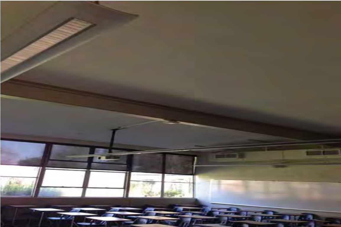
Photograph 3-General view of the interior suspect building materials
