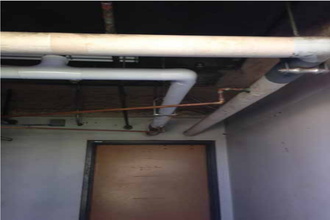
Photograph 11-View of the suspect pipe insulation materials
