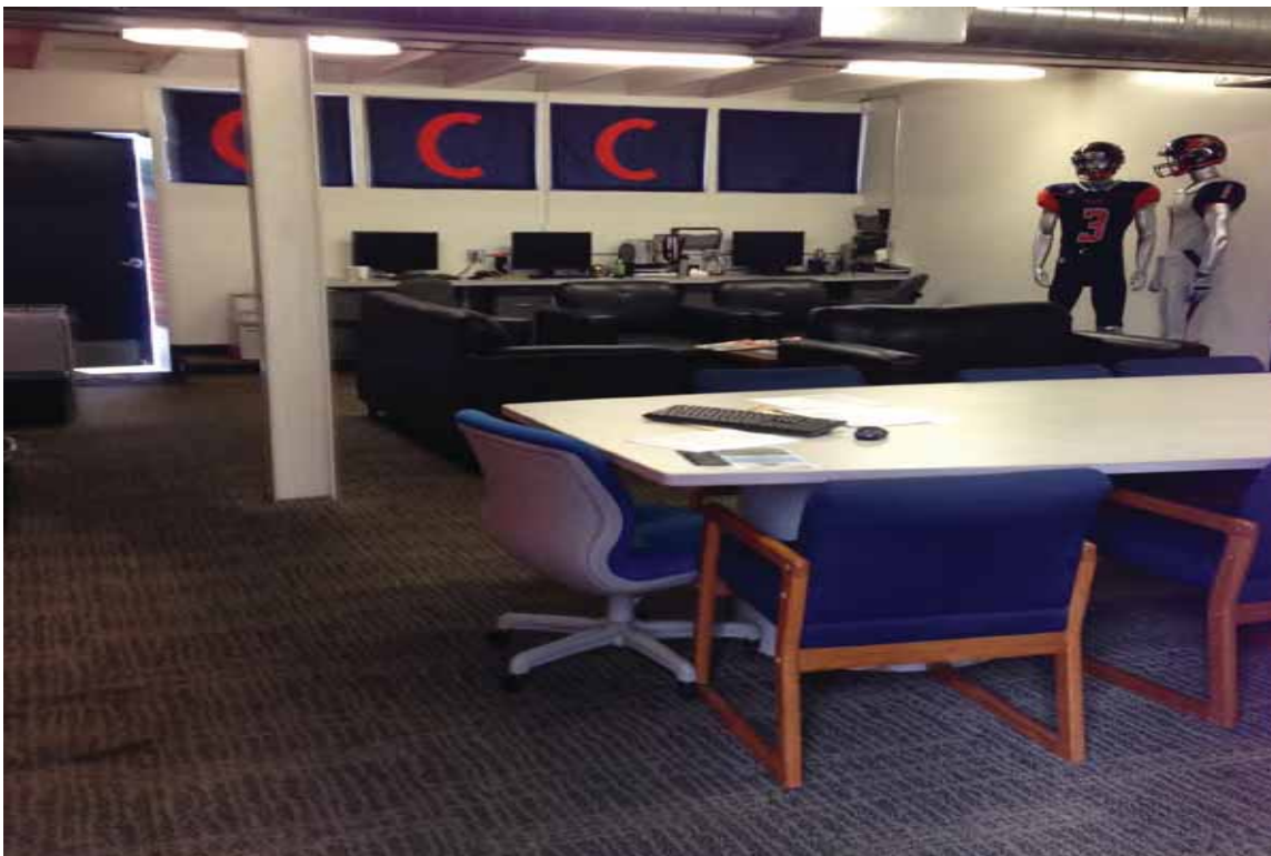
Photograph 6-General view of the suspect interior building materials, Including ACM, lead paint, ballasts and mercury light bulbs
