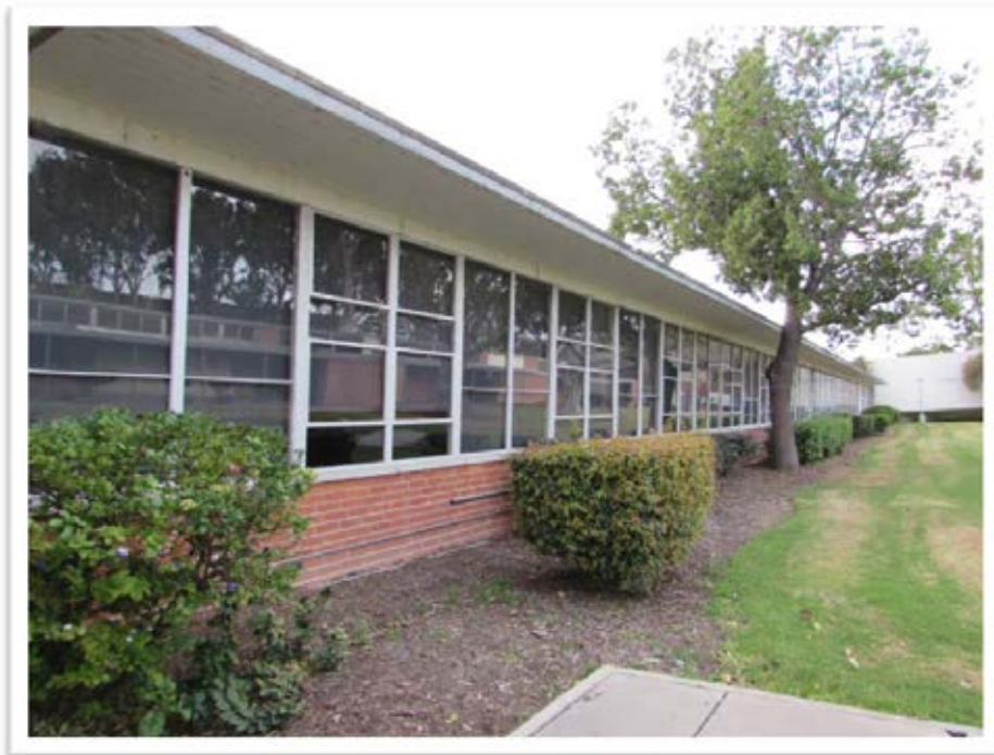
PHOTO - 38: Classroom wing fenestration and canopy overhang details, 2014.
