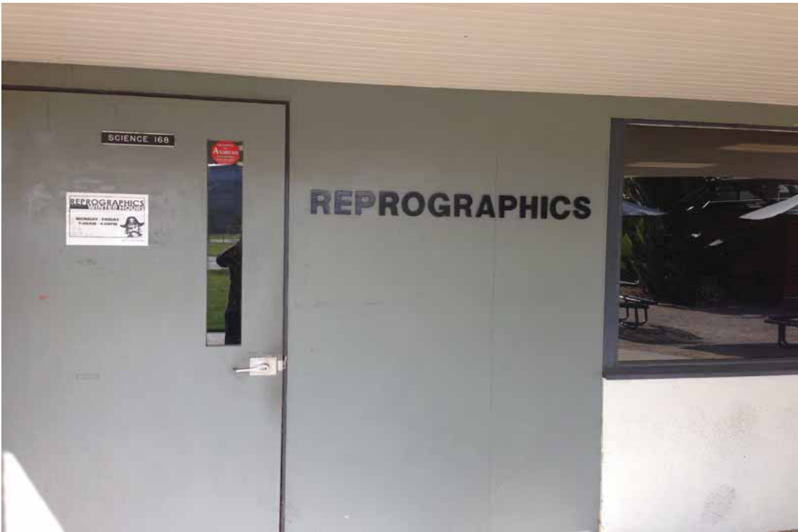
Photograph 9-General front view of the building 37
