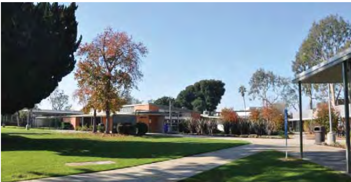
Figure 1C-116: Journalism (Bldg. 72, 1958) and Writer's Row (Bldg. 71, 1958, right) adjacent to the northwest corner of Historic District boundaries, looking northwest.
