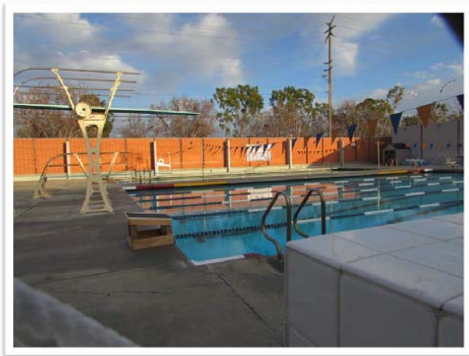
PHOTO - 30: Swimming pool stadium, looking east, 2014.
