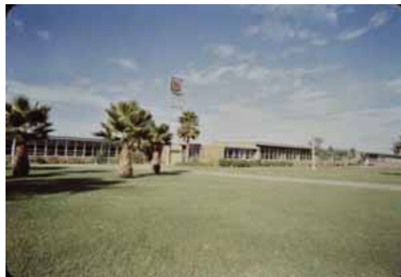
Figure 1B-21: Facing south towards Building 7 (left-hand side) and Buildings 8 & 9 (right-hand side). Date unknown. Source: Box 99, Robert Evans Alexander papers, #3087. Division of Rare and Manuscript Collections, Cornell University Library.
