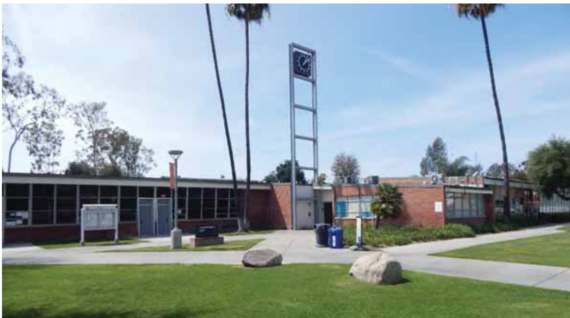
Figure 1: Student Success Center and Classroom & Labs complex (Bldgs. 7 -9), 3
