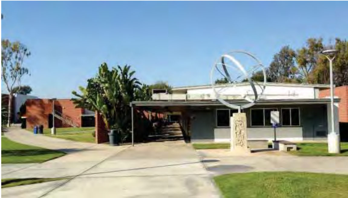
Figure 161: East façades of Building 35, left, and 37, left background, looking west.
