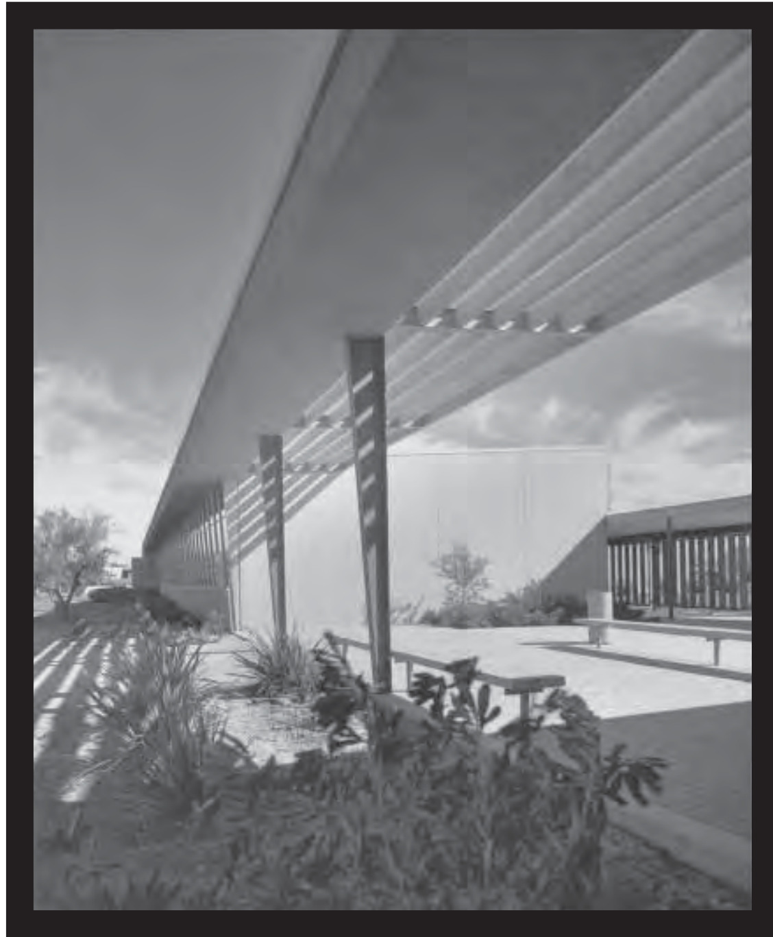
North elevation of Library Addition (Classroom and Lab, Bldg. 8). Julius Shulman Photography Archive. Copyright The J. Paul Getty Trust. The Getty Research Institute, Los Angeles.
