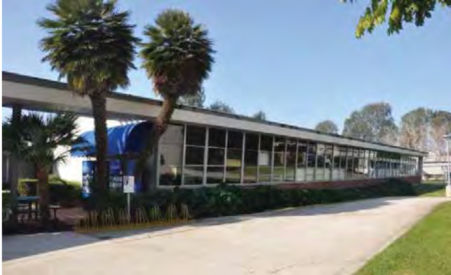
Figure 1C-18: Building 9's north façade with typical windows.
