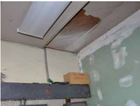
Figure 247: Partial repairs undertaken in mechanical room, Field House, Building 110.
