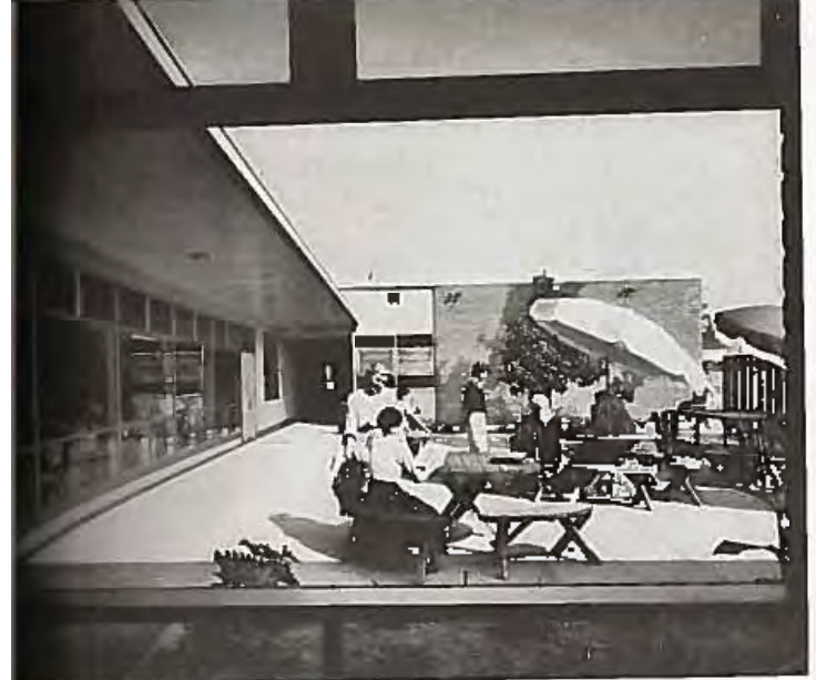
Open sliding doors join lounge and main dining room (right). Structure is basically wood frame on concrete slab, grade beams, and coissons. Exterior materials include plaster, brick, and enameled-metal sunshades. Floorings are wood block or asphalt tile; acoustical tile is used on ceilings. Sash is aluminum-primed type. Parker, Zehnder & Associates, Structural Engineers; Bartlett & Berky, Mechanical Engineers; Sheldon W. Swickard, Electrical Engineer.
