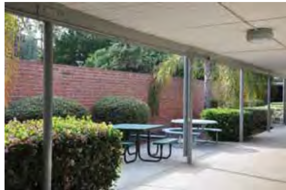
Figure 1C-28: Brick screen wall with concrete slab and planting strips south of Bldg. 9's south covered walkway, looking west.
