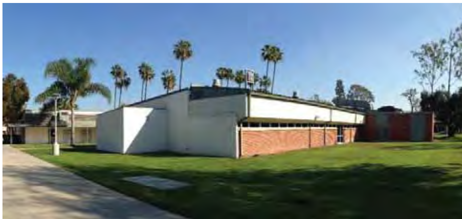
Figure 1C-9: Building 7's west wing with its brick-clad and stucco fascia south façade and tilt-up concrete wall west façade and shed addition. Standing seam metal roof on the south half of the building visible.
