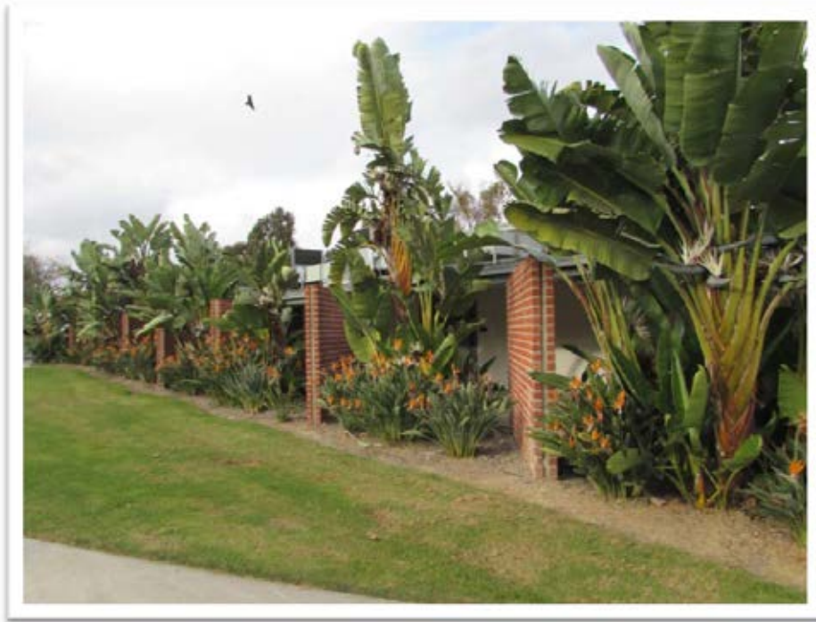
PHOTO - 13: Windbreak walls with landscaping along corridor of Science Building (aka Math Wing), looking northeast, 2014.
