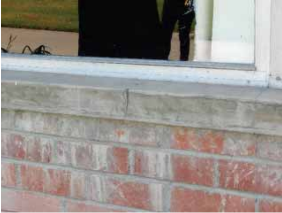
Figure 102: Cement slurry coating brickwork below concrete sill.
