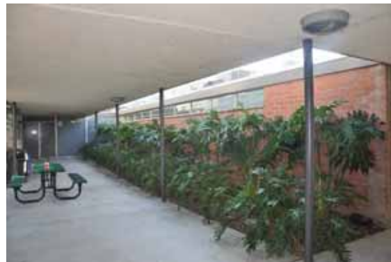
Figure 1C-50: Brick-clad L-shaped wing at the southwest corner of the Theater Building. Looking east.
