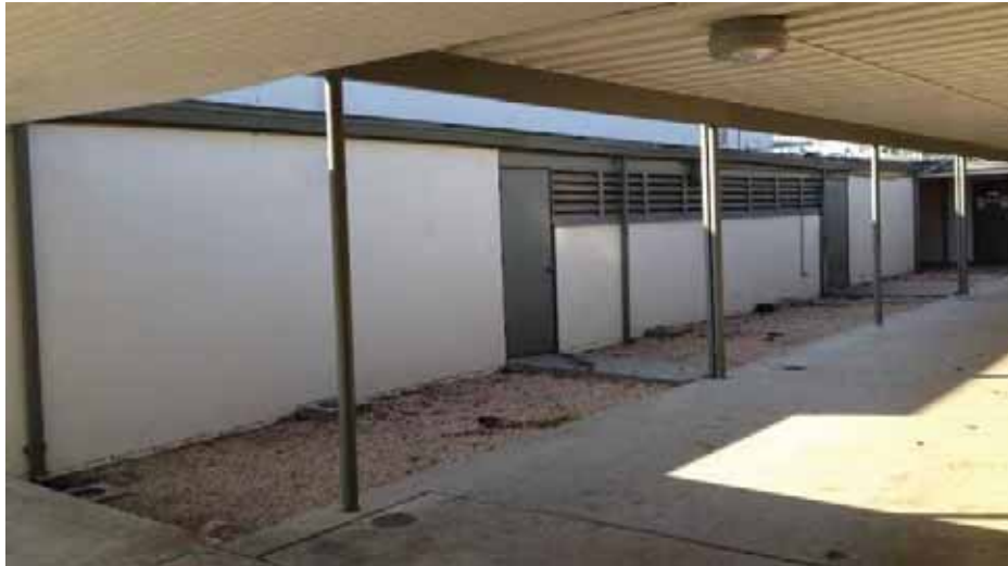
Figure 1C-77: Building 37's north façade along the covered walkway.
