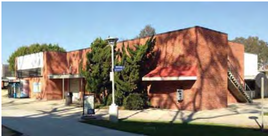
Figure 1C-76: South façade of Building 37. At the right is the east façade with exterior stairs to the roof-top observation deck.
