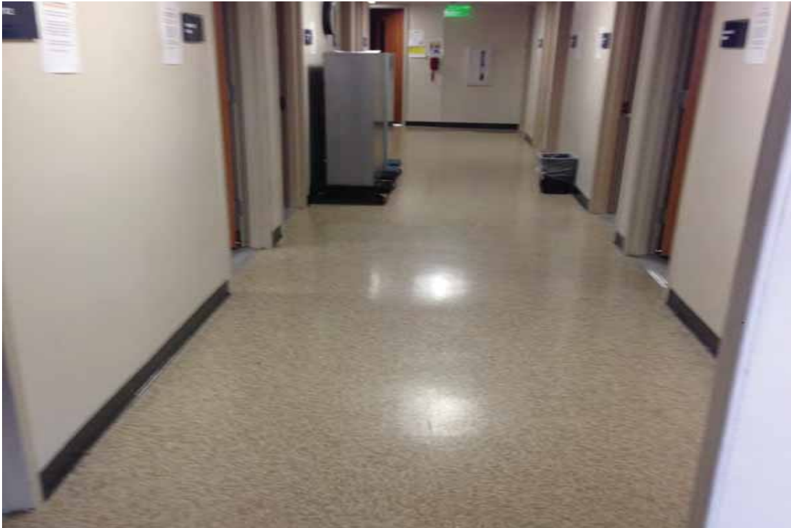
Photograph 13-General view of the interior suspect building materials
