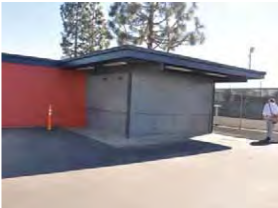
Figure 1C-109: Concession area on the west façade, looking east.
