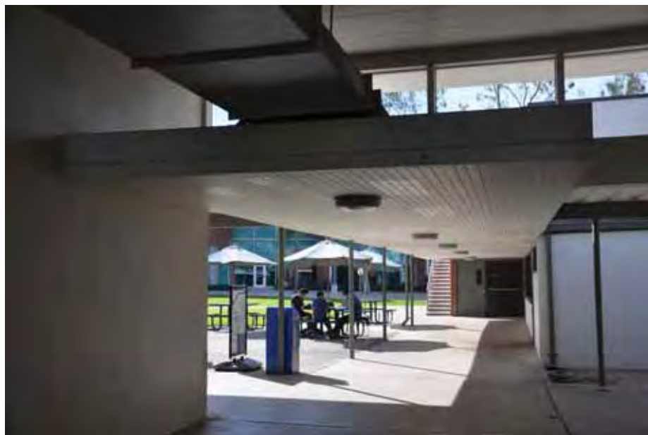
Figure 1B-36: Breezeway between Building 35 and 36 with HVAC duct added and louvers removed.
