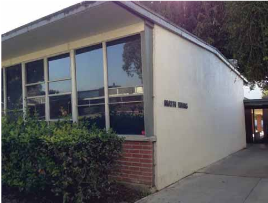
Figure 1C-69: Building 36's west end wall with the tapered aluminum section transitioning to the building's angled north glazed wall.
