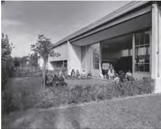
Figure 1A-12: Outdoor classroom space with sliding glass walls at Corona Avenue School, ca.1953. Julius Shulman Photography Archive. Copyright The J. Paul Getty Trust. The Getty Research Institute, Los Angeles. ID no.: gri_2004_r_10_b0079_f012_1545_04.
