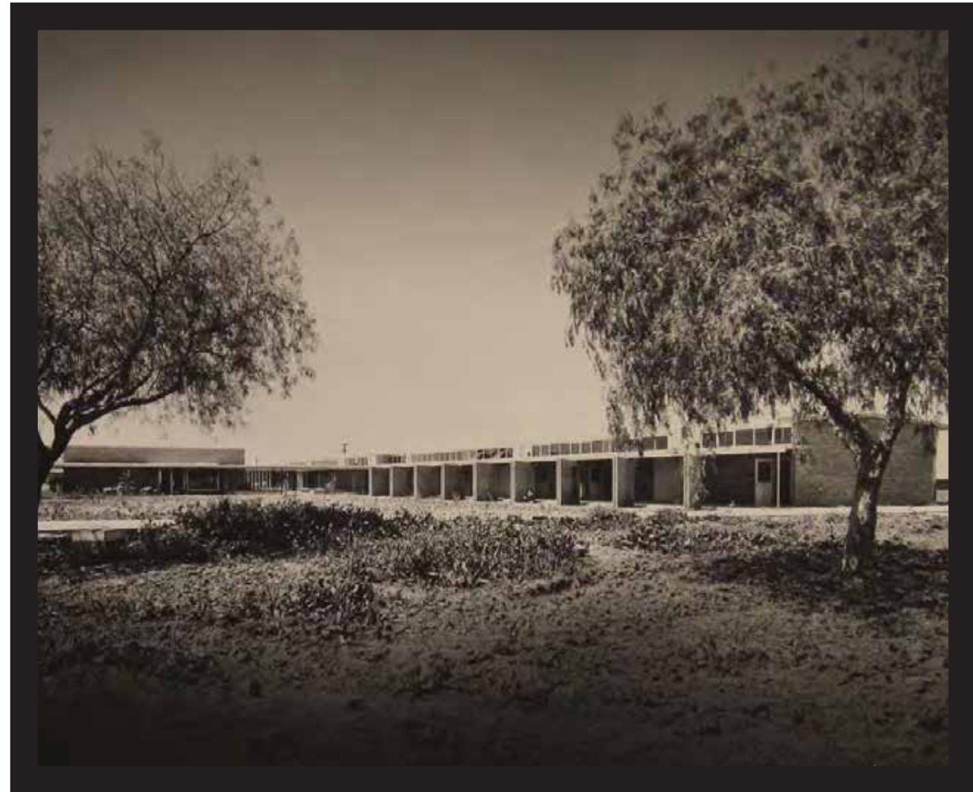
South elevation of the Business Education (Business Education, Bldg. 12, 13, and 14); ca. 1954 by Julius Shulman. Source: Robert E. Alexander Collection, Division of Rare and Manuscript Collections, Cornell University Library.
