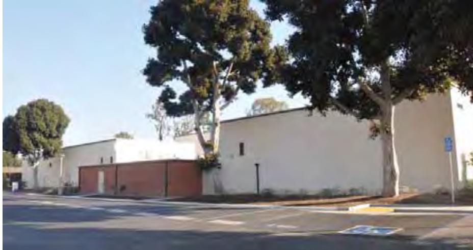
Figure 1C-59: West façade of Building 4 (left) with the brick-clad section centered.
