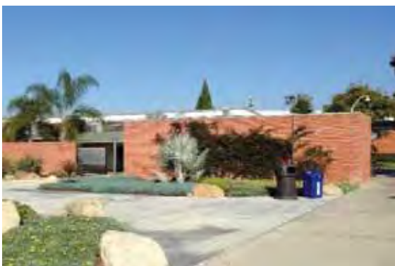
Figure 1C-22: Building 9b's south facades with adjacent brick screen wall, looking northwest.
