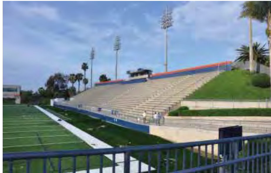
Figure 30: Building 105 LeBard Stadium, 2015. Source: Page & Turnbull.
