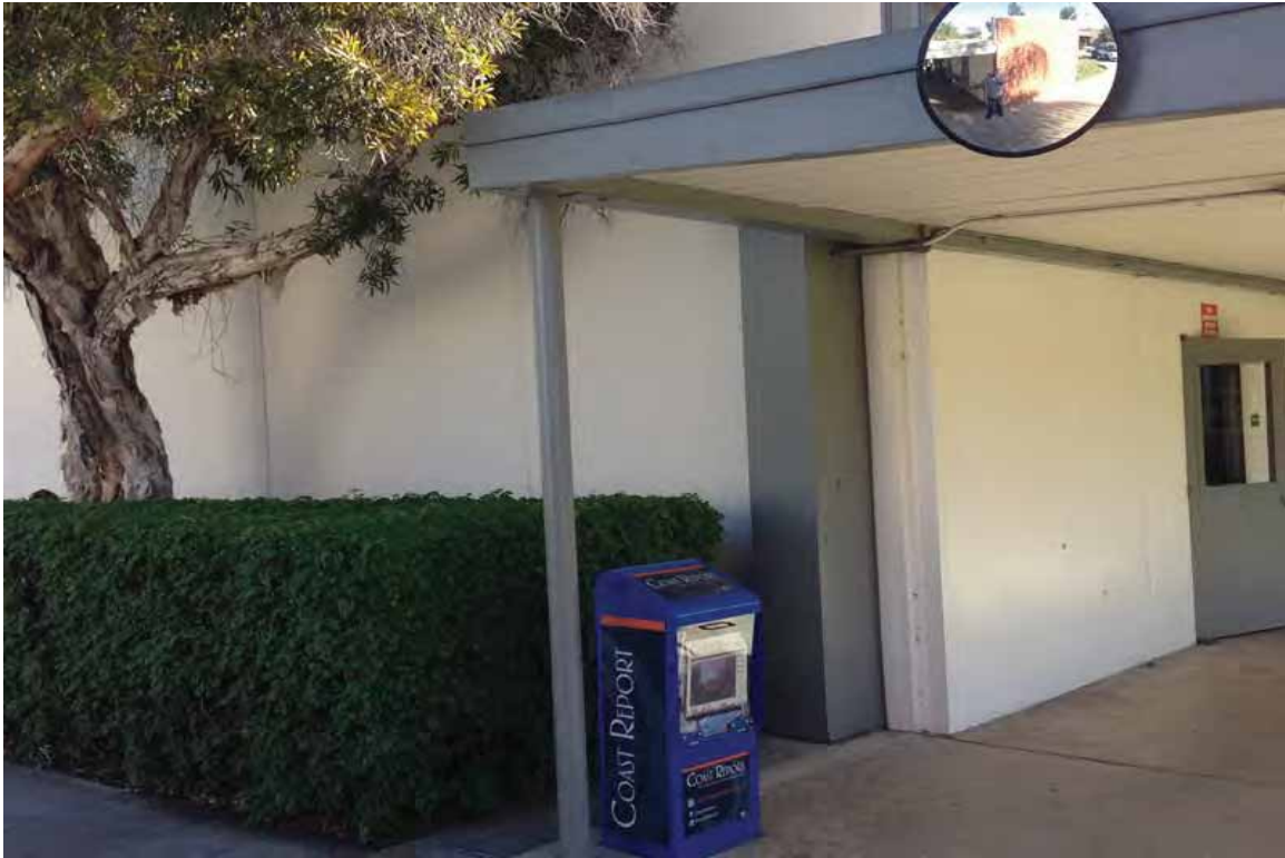
Photograph 1-General front view of the subject buildings
