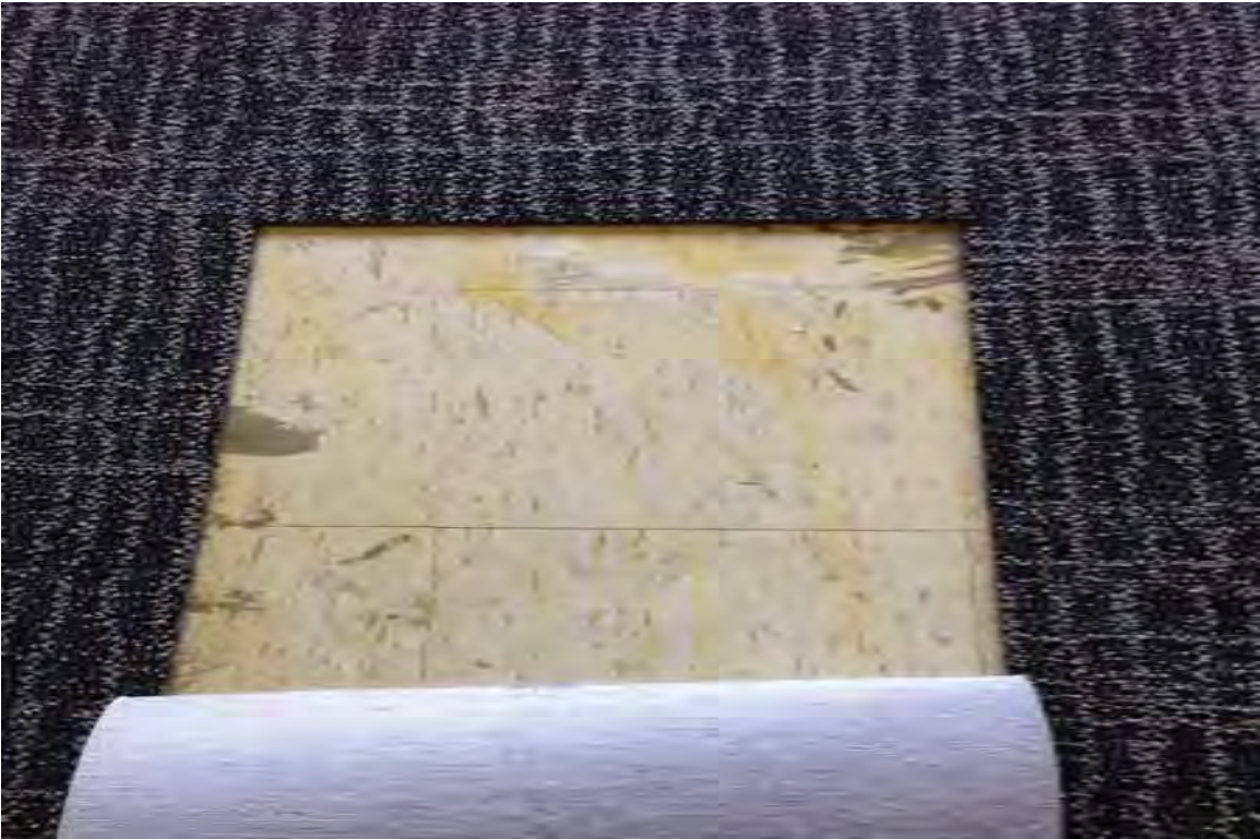
Photograph 5-View of the suspect flooring materials under carpet
