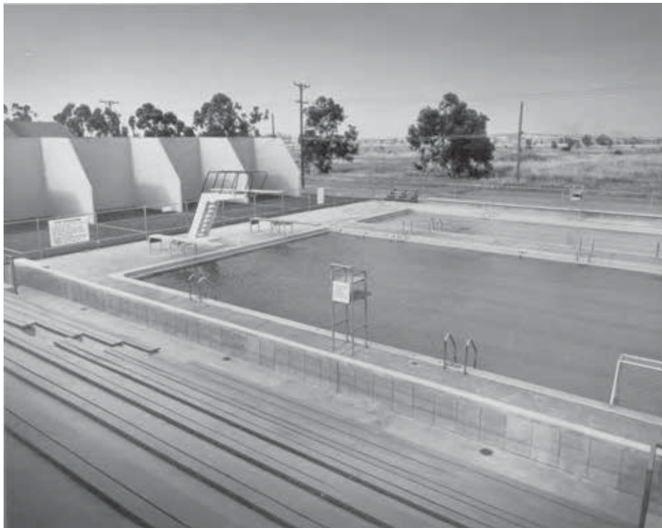
Figure 1B-40: View of the swimming pools from the bleachers facing northeast. The handball courts in the background have been demolished and the Men's Locker Room (Bldg. 96) constructed in its place. Date unknown. Julius Shulman Photography Archive. Copyright The J. Paul Getty Trust. The Getty Research Institute, Los Angeles. ID no.: gri_2004_r_10_b0080_f001_1745_33.
