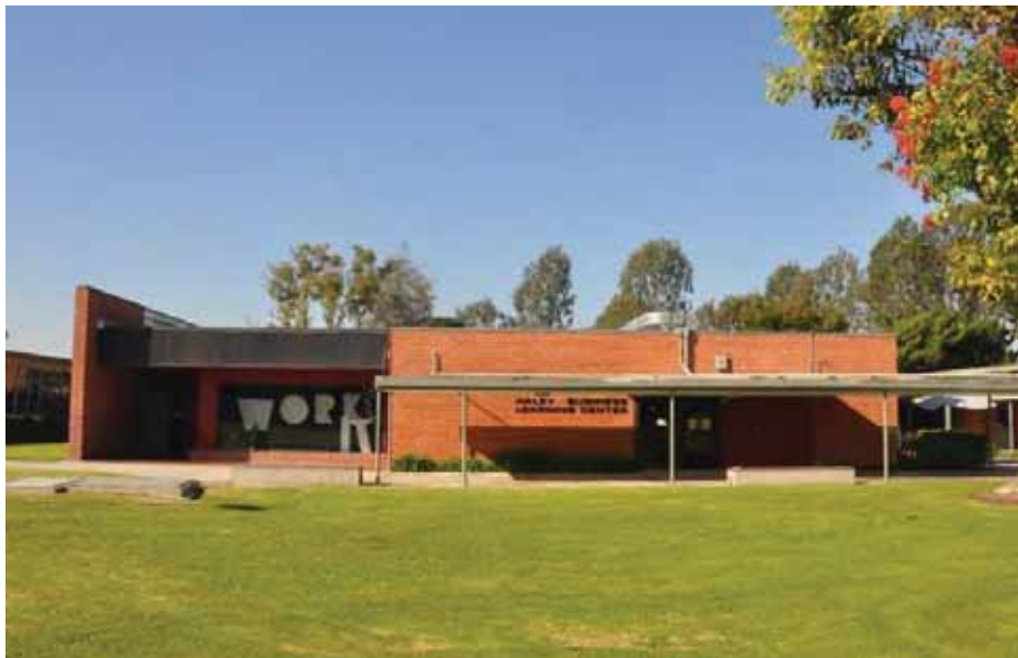
Figure 1C-38: East façade of Building 14, looking west. Building 12 and 13 are to the right (north). The right brick façade is the original building before an addition (left) was added in the 1970s.
