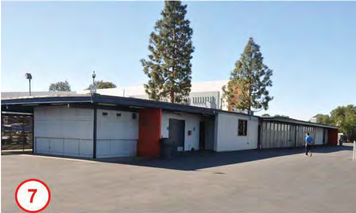
Figure 1D-37: Contemporary image of the Field House (Bldg. 110) with character defining features identified by red callouts.
