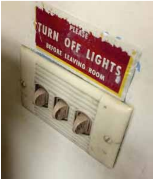
Existing light switches
