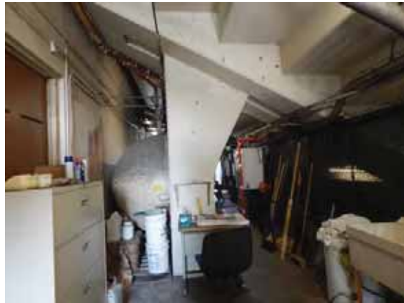
Figure 1C-100: Sculptural concrete pier in the mechanical room below the bleachers.
