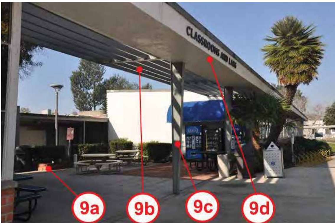
Figure 1D-9: Contemporary image of the Student Success Center and Classroom & Labs (Bldgs. 8 & 9 in photograph) with character defining features identified by red callouts.
