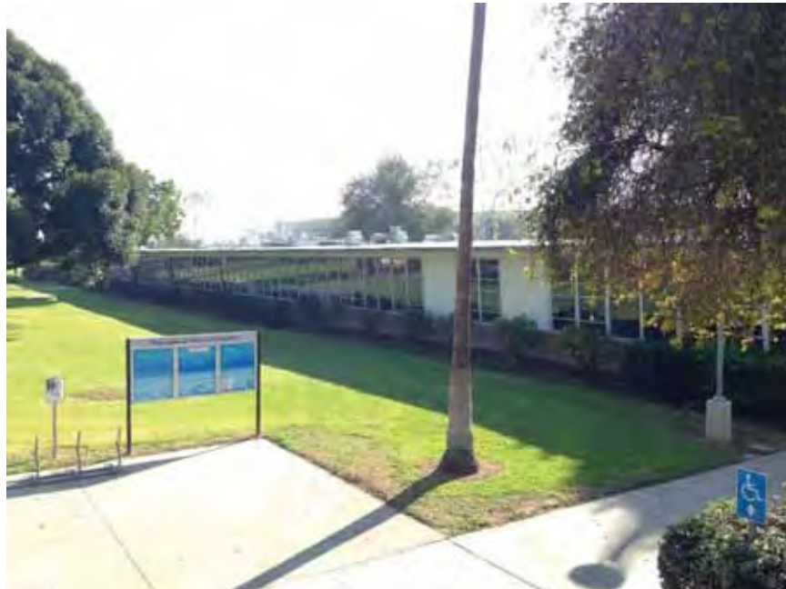
Figure 1B-38: North façade of Building 36 with 1960 addition with stucco bays.
