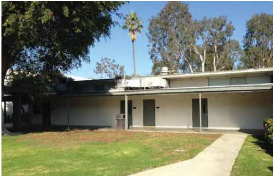
Figure 1C-70: Typical south façade of Building 36 showing the clerestory windows, stucco panels and HVAC units mounted on the walkway canopy.
