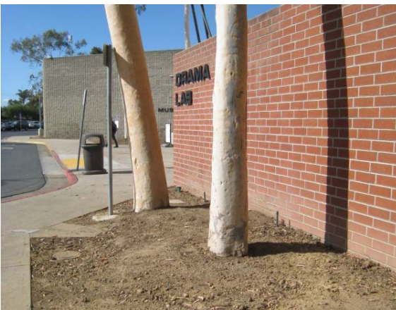
Figure 5. View north toward Drama Lab from the parking lot in the southeastern portion of the campus.
