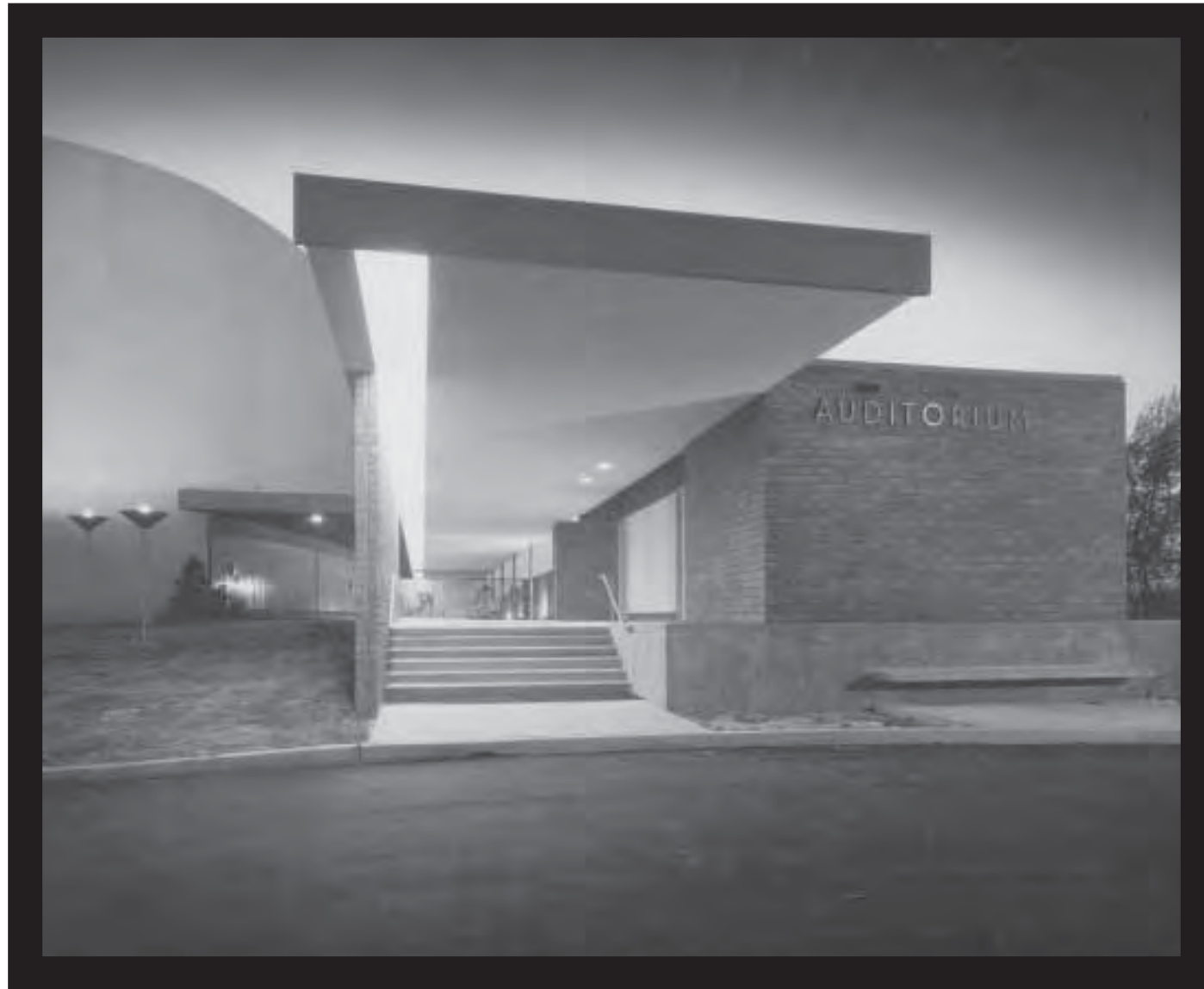
East elevation of the Theater Box Office (Robert Moore Theater, Bldg. 2); ca. 1955. Julius Shulman Photography Archive. Copyright The J. Paul Getty Trust. The Getty Research Institute, Los Angeles.
