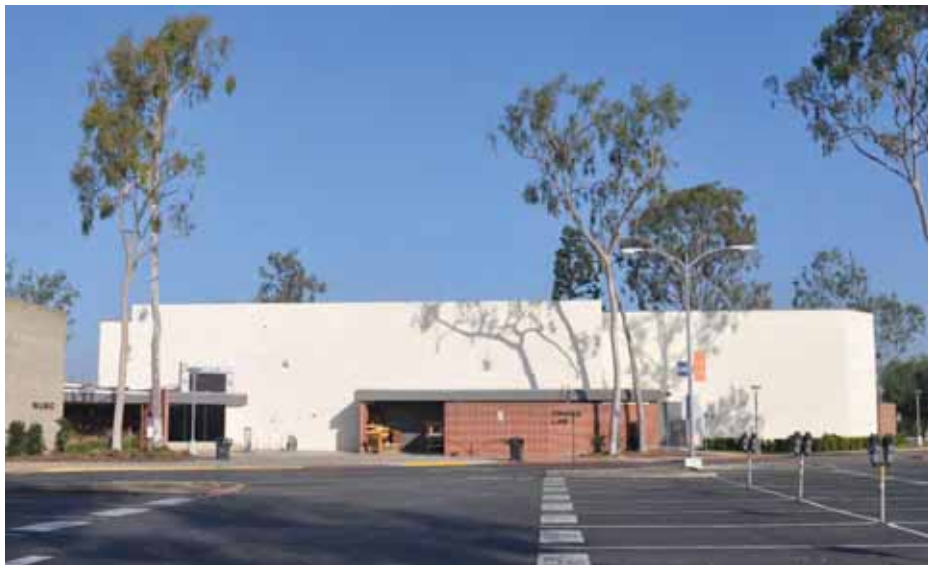
Figure 1C-48: Rear of the Moore Theater, which is the Drama Workshop addition from the 1970s. The triangular entrance to the second performance space is at left, as is Building 3, also from the 1970s. Looking north.
