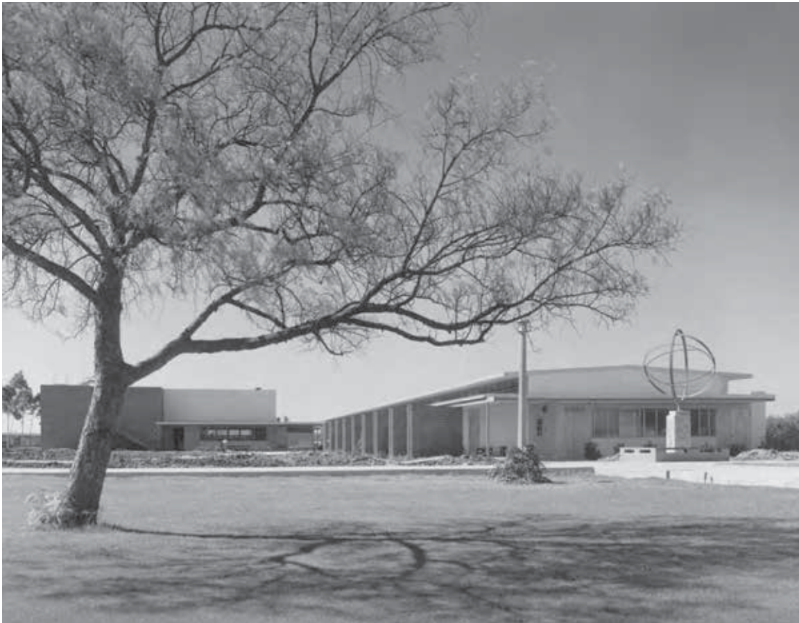
Figure 1D-23: Historic image of the Math & Planetarium complex (Bldg. 35-39). Photo by Julius Shulman, 1957, Getty Research Institute.
