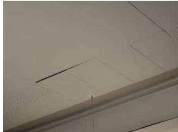
Figure 185: Detaching ceiling tile with no visible water damage at Building 36.
