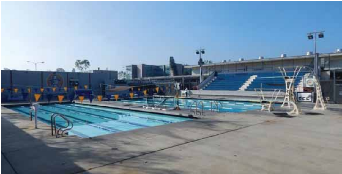
Figure 5: Swimming Pool complex (Bldg. 93).
