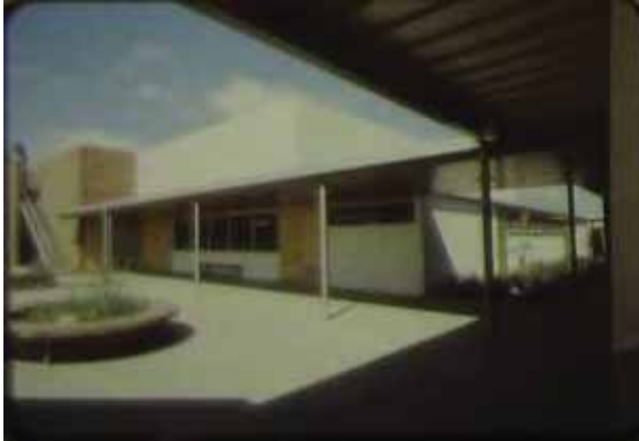
Figure 1B-33: Historic photograph of the east façade of Building 37 showing exposed plywood with clear finish (low resolution image). ca. 1957. Source: Box 99, Robert Evans Alexander papers, #3087. Division of Rare and Manuscript Collections, Cornell University Library.
