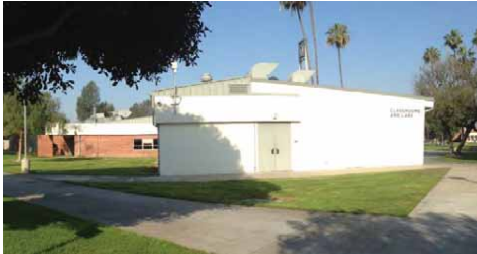
Figure 1C-8: Building 7's concrete east façade (east wing) with the west wing's brick east façade and recessed rear south entrance in the background, looking northwest. The building's original shed and flat roof outline is visible above the east façade, as is the added standing seam metal roof on the south half of the building.
