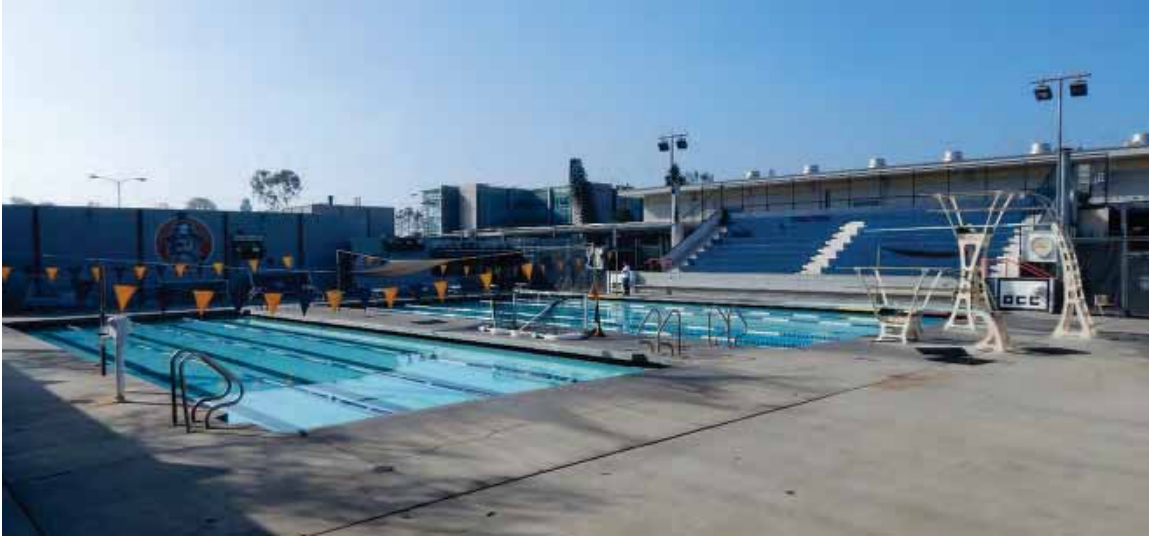
Figure 192: Swimming Pool complex (Bldg. 93), facing southwest.
