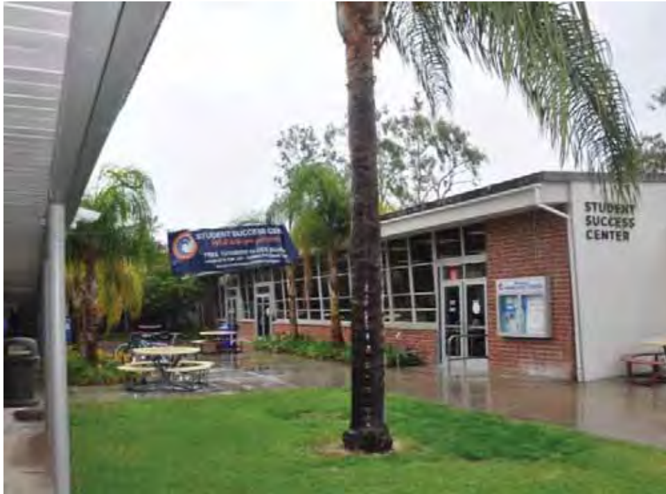
Figure 1C-5: North window wall façade of Student Success Center (Bldg. 7) west wing looking east to the building's north elbow.
