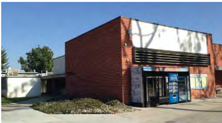
Figure 1C-80: West (left) and south (right) façade of Building 37. Note the aluminum louvers screening clerestory windows on the south façade. The stucco south façade of Building 38 is also visible at the left.
