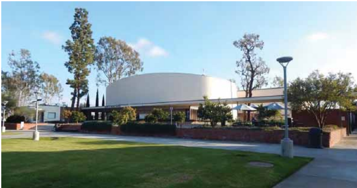
Figure 1C-42: The Theater and Music complex with the Robert B. Moore Theater (Bldg. 2) and its outdoor lobby below the covered walkway. The Music Building (Bldg. 4) is out of frame to the right. Looking southeast.
