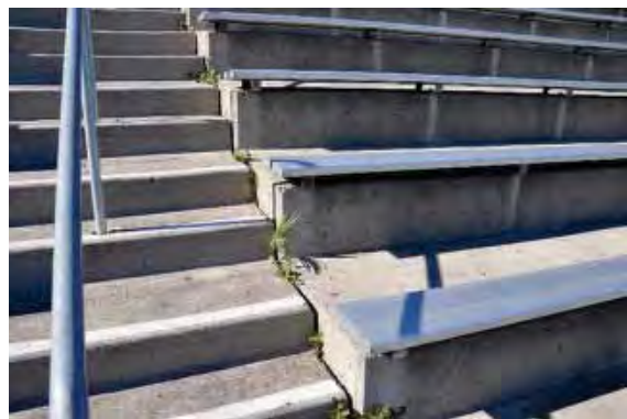
Figure 227: Plant growth in a crevice at the side of the steps on the west bleachers.
