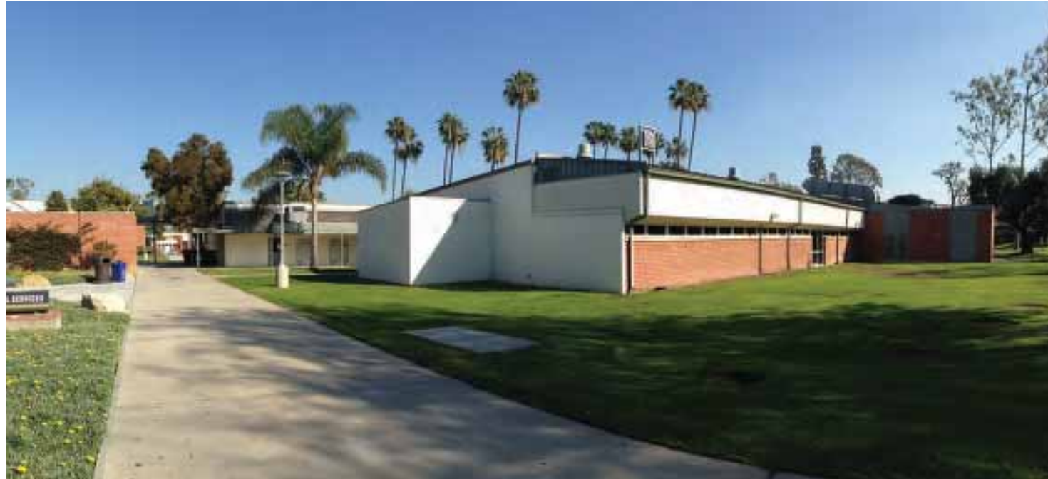
Figure 9: View of Building 8 and additions to Building 7, 2015. Source: Page & Turnbull.
