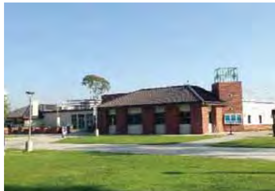
Figure 1B-15: Current Student Center (Bldg. 86) after 1990s alteration. 40
