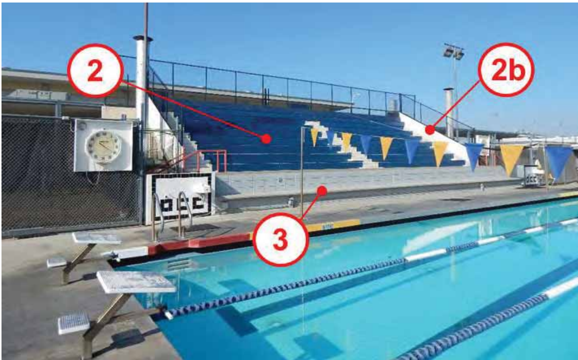
Figure 1D-31: Contemporary image of the Swimming Pool complex (Bldg. 93) with character defining features identified by red callouts.
