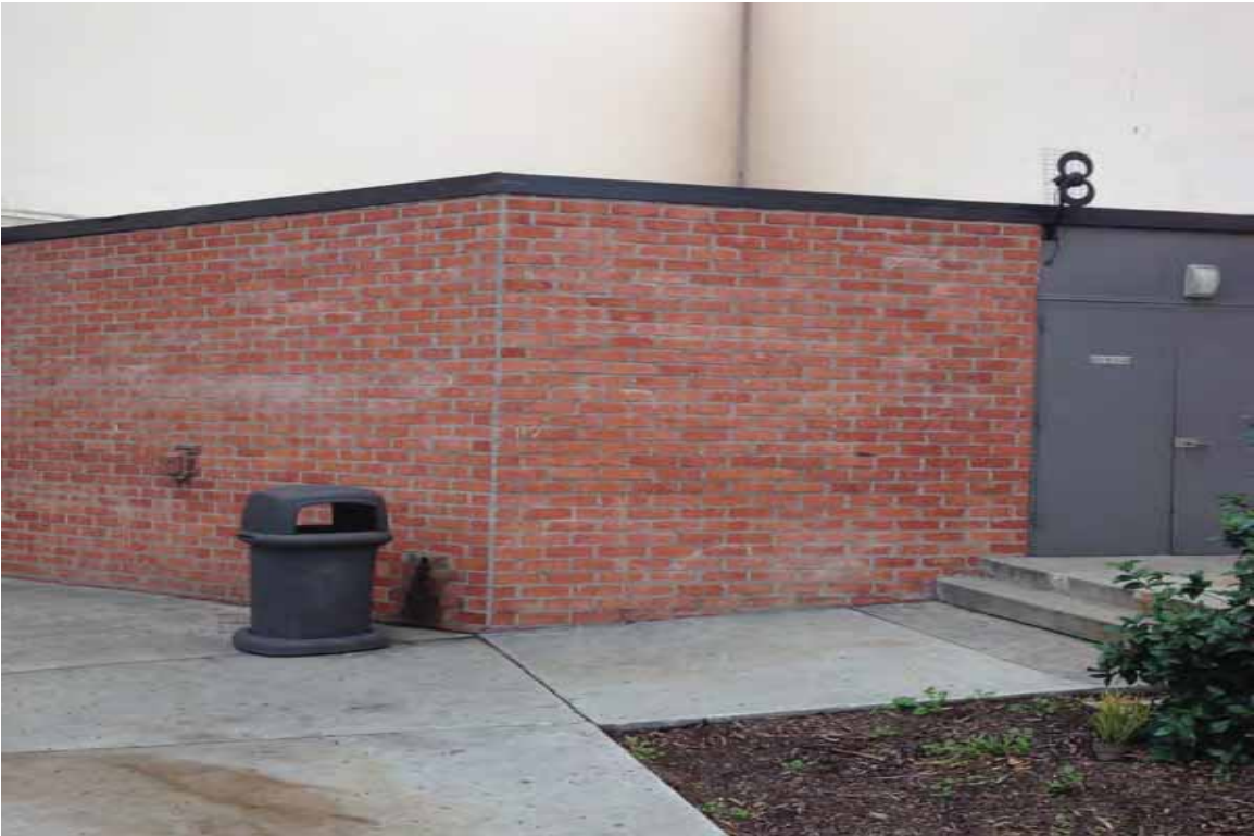
Photograph 7-General exterior view of the exterior
