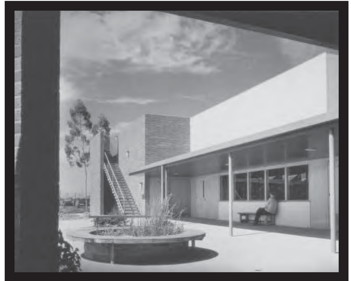
South elevation of the Laboratory Building (Reprographics, Bldg. 37); ca. 1957. Julius Shulman Photography Archive. Copyright The J. Paul Getty Trust. The Getty Research Institute, Los Angeles.
