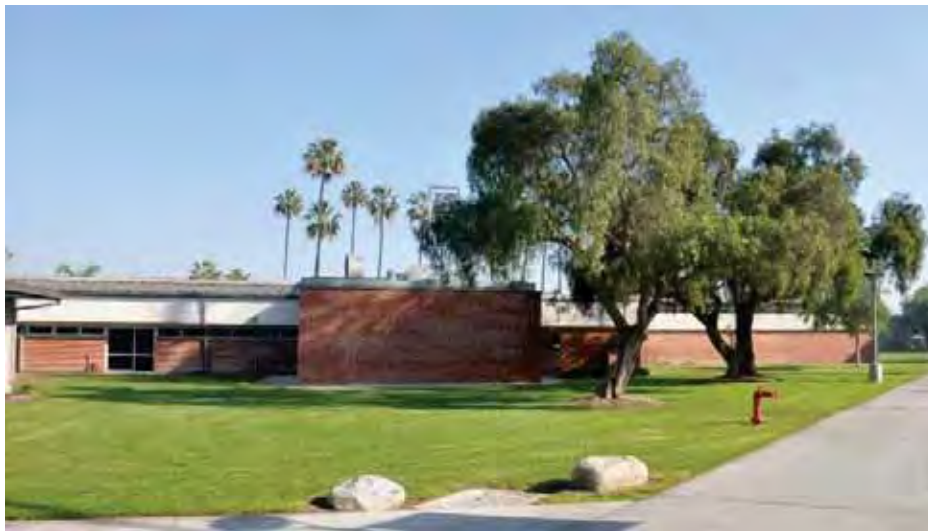
Figure 1C-7: South façade of Building 7 with west wing to the left, mechanical room addition in center, and east wing to the right, looking plan north.
