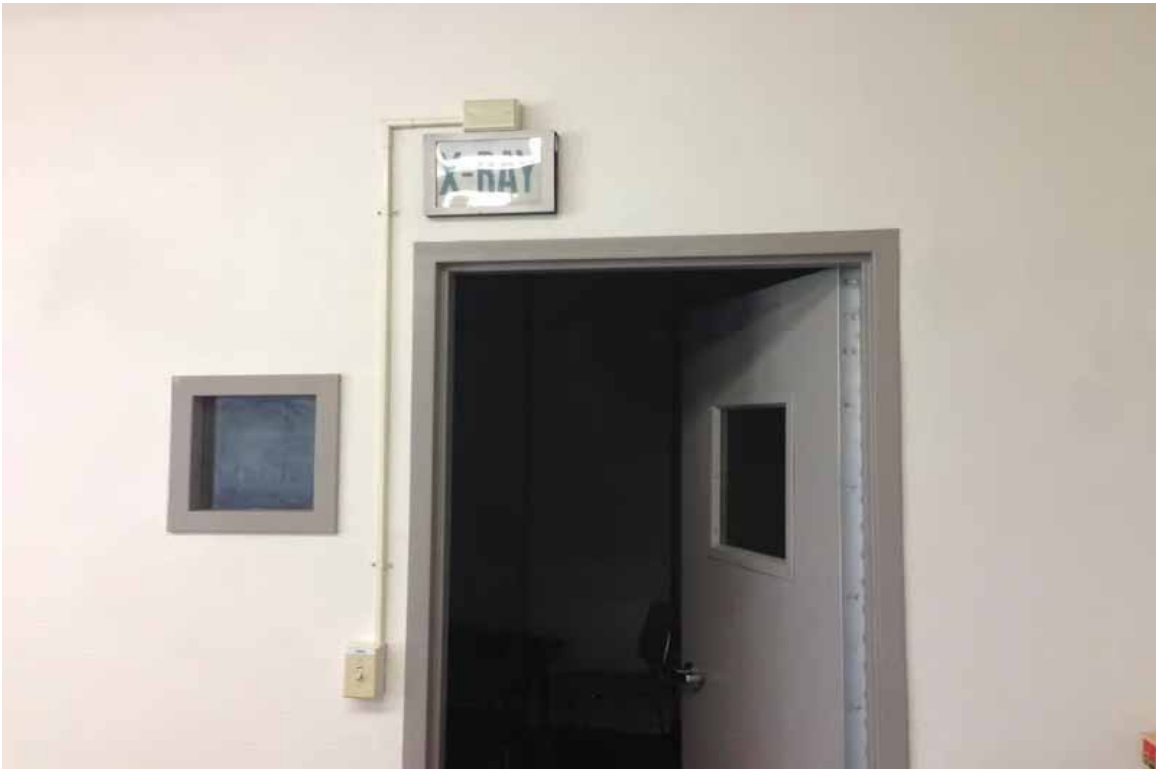
Photograph 10-View of the suspect lead-containing materials in the X-Ray room
