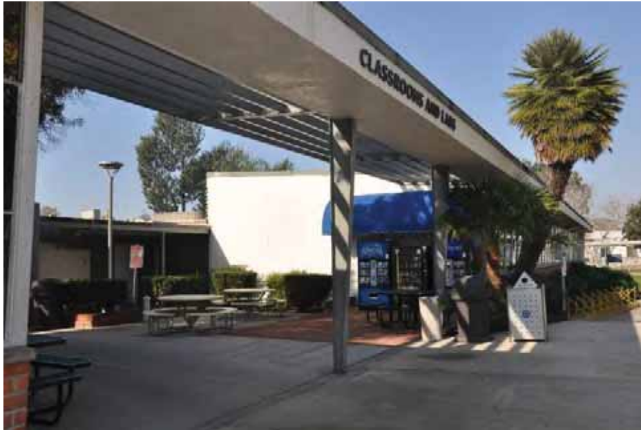
Figure 1C-26: Landscaped patio with brick and concrete paving and a low L-shaped brick planter between Buildings 8 and 9. Note the trellis, soffit, and support posts.
