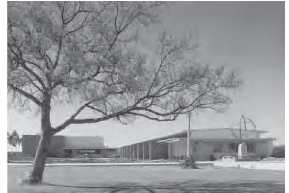
Figure 21: Buildings 35 & 37 Math & Reprographics, ca.1957. Source: Julius Shulman Photography Archive. Copyright The J. Paul Getty Trust. The Getty Research Institute, Los Angeles. ID no.: gri_2004_r_10_b0082_f012_13_2453_01.
