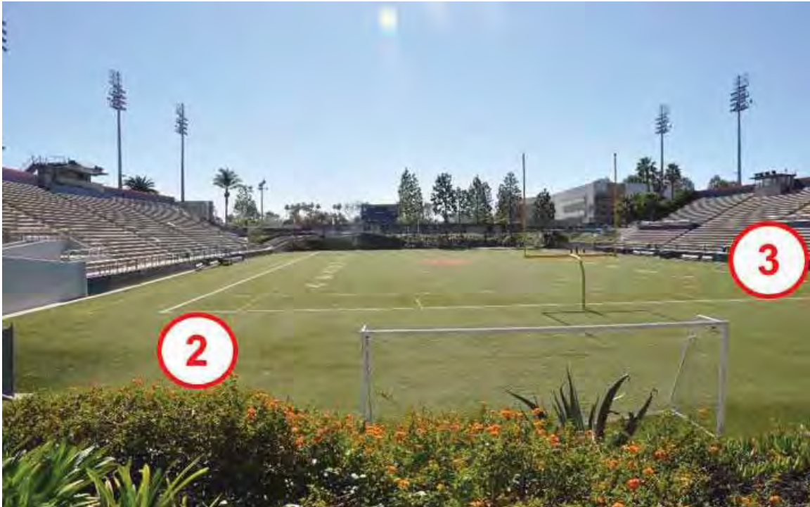
Figure 1D-35: Contemporary image of the Stadium and Field House (Bldg. 105 & 110) with character defining features identified by red callouts.
