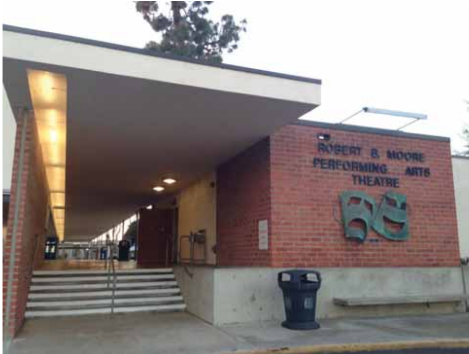
Figure 1C-54: Building 2B at right and the Moore Theater (Bldg. 2) is at left. Note the integrated strip of lighting in the covered walkway connecting the two buildings. Looking west from circular drop-off driveway.
