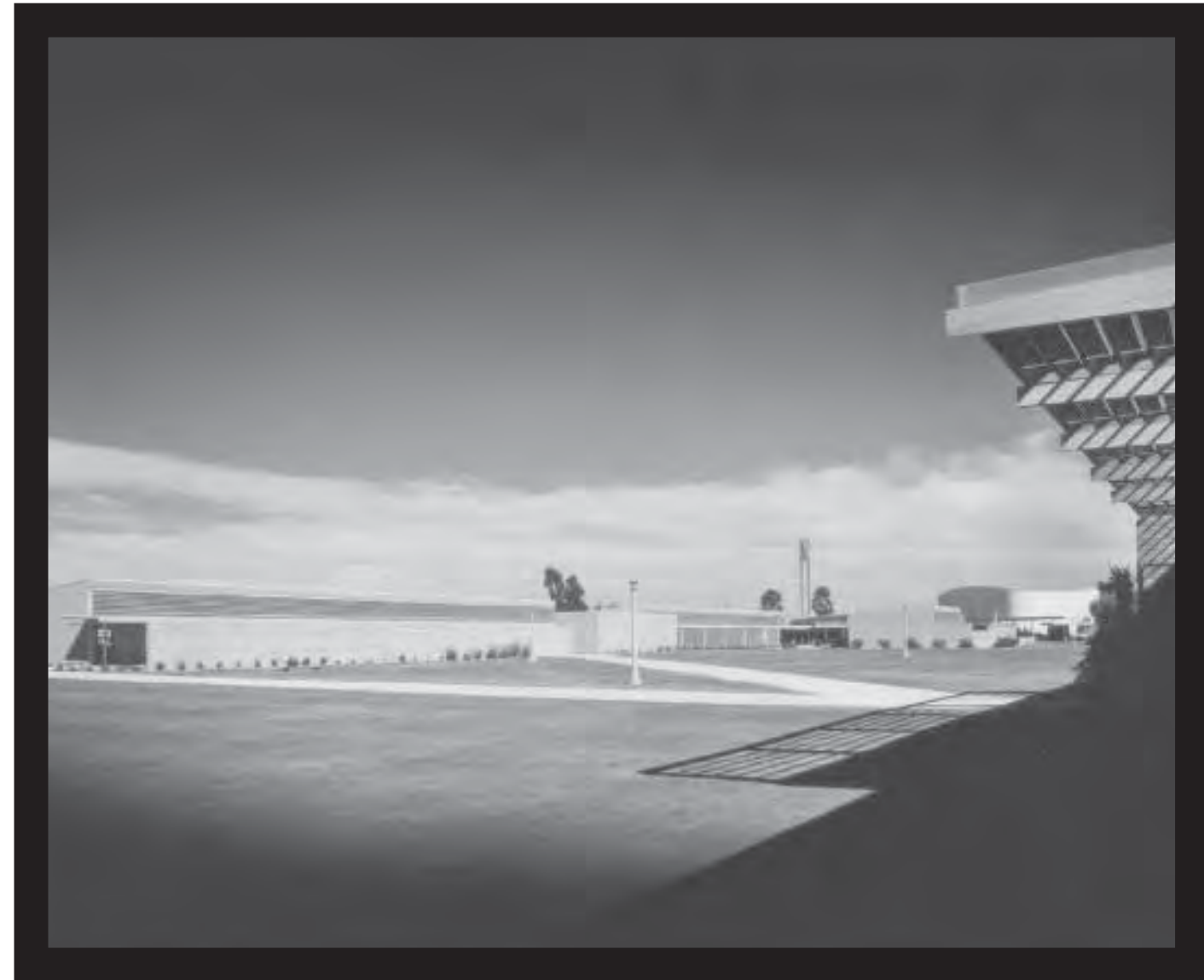
West elevation of Library and Classroom additions (Student Success Center, Classroom and Labs, Bldg. 7, 8, and 9). Julius Shulman Photography Archive. Copyright The J. Paul Getty Trust. The Getty Research Institute, Los Angeles.
