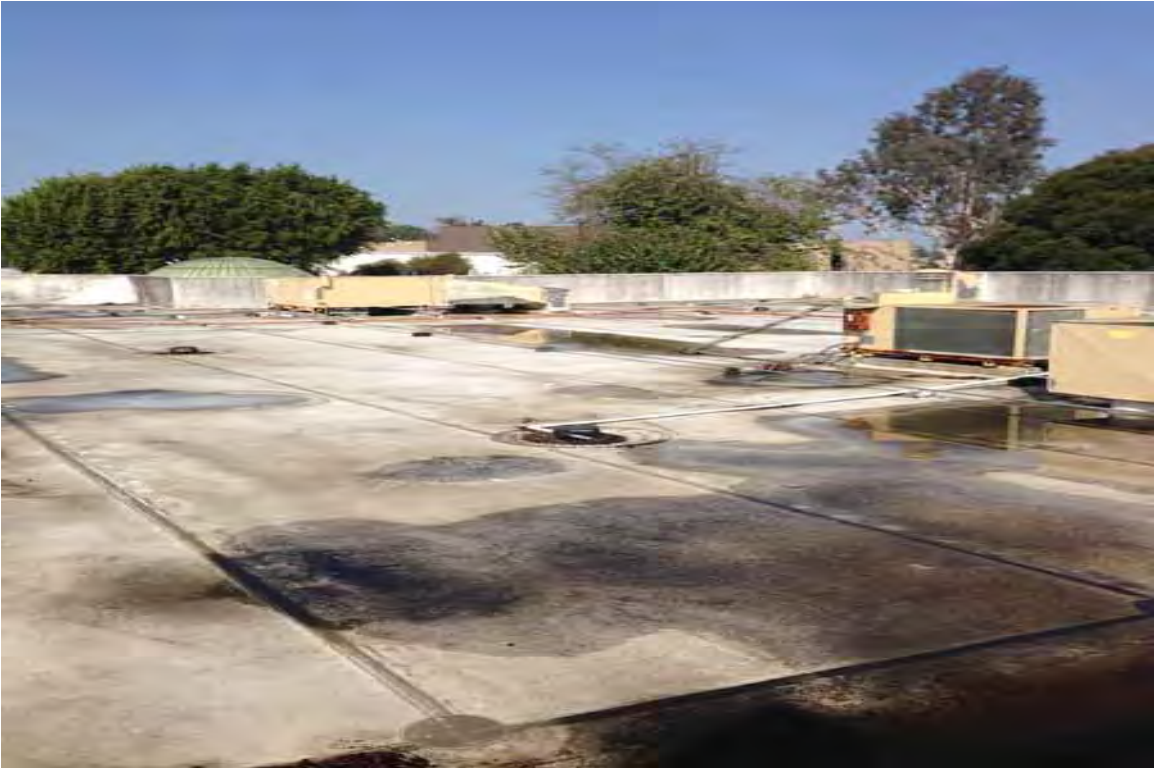
Photographs 18-General view of the suspect roofing materials
