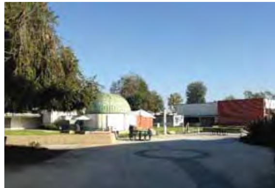
Figure 1C-95: Open space surrounding the Planetarium (Bldg. 39) with the Reprographic Building (Bldg. 37) at right, looking southeast.
