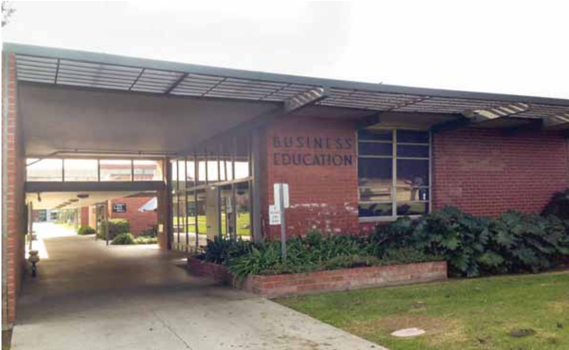
Figure 1C-29: Business Education breezeway between Bldg. 12 (left) and Bldg. 13 (right), looking south to Bldg. 14.
