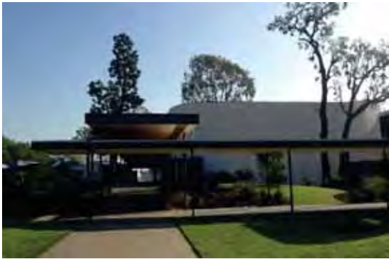
Figure 1C-64: West end of terrace with overlapping covered walkways and lawn to the south.
