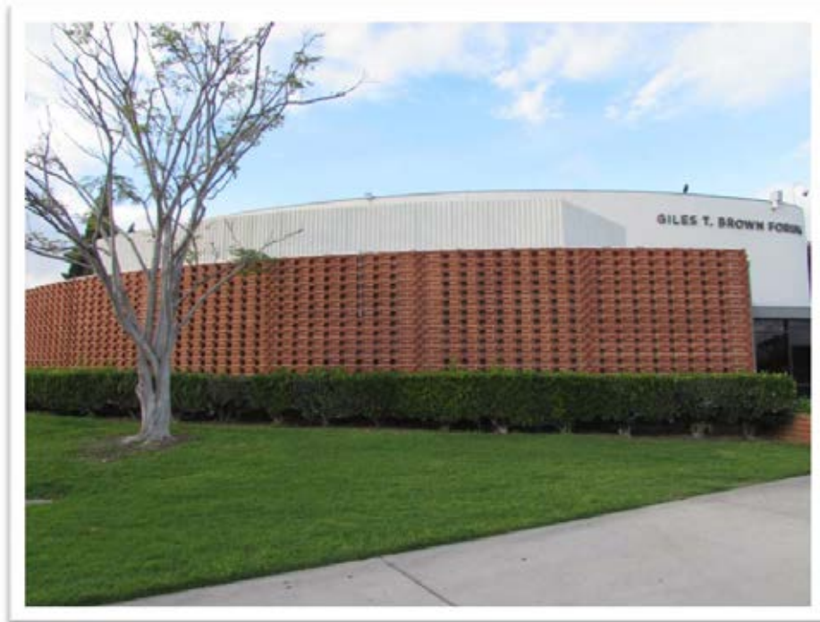
PHOTO - 20: Social Science Forum façade, looking north, 2014.
