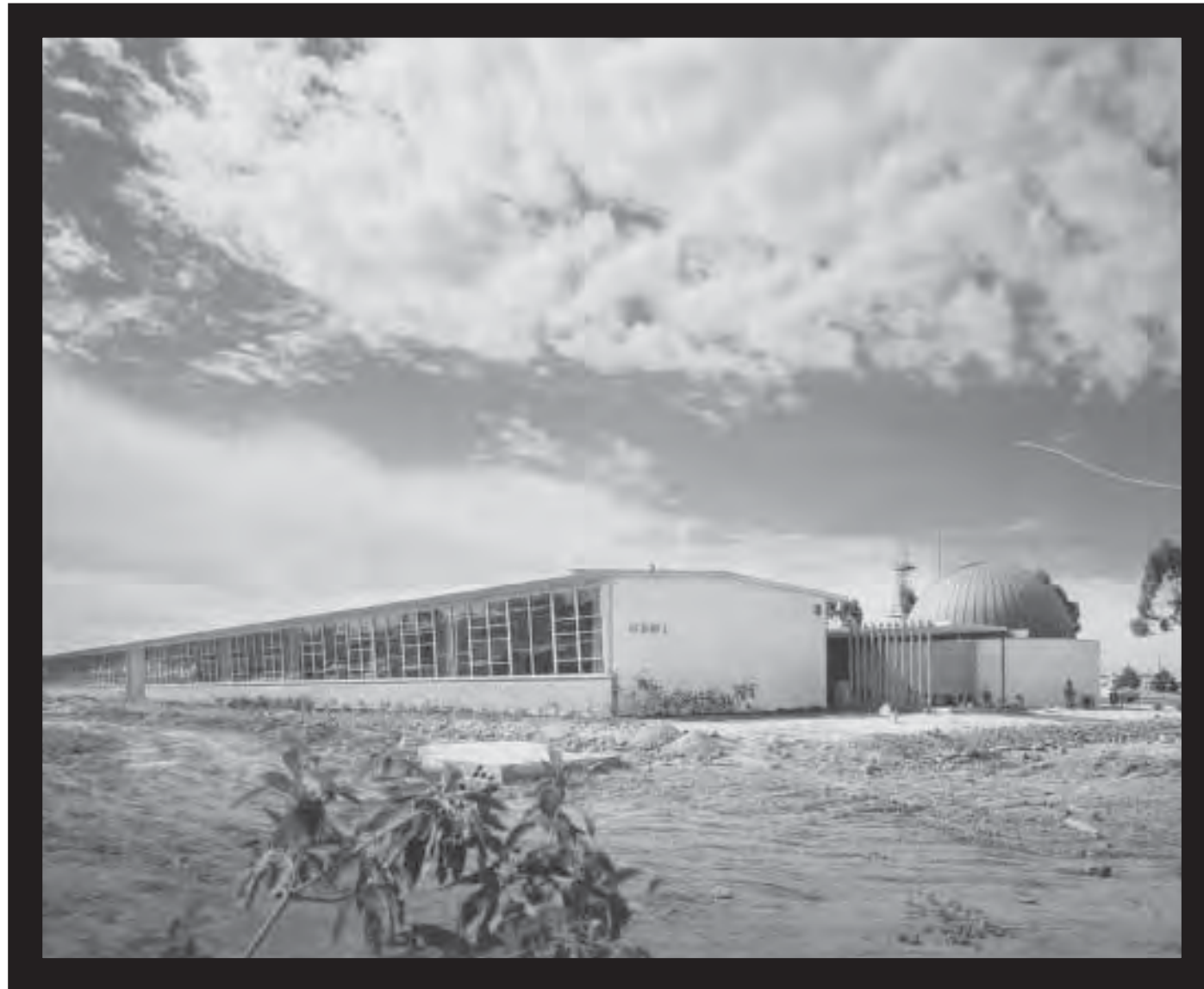
North elevation of the Science Building (Math Wings and Planetarium, Bldgs. 35, 36, and 39); ca. 1957. Julius Shulman Photography Archive. Copyright The J. Paul Getty Trust. The Getty Research Institute, Los Angeles.
