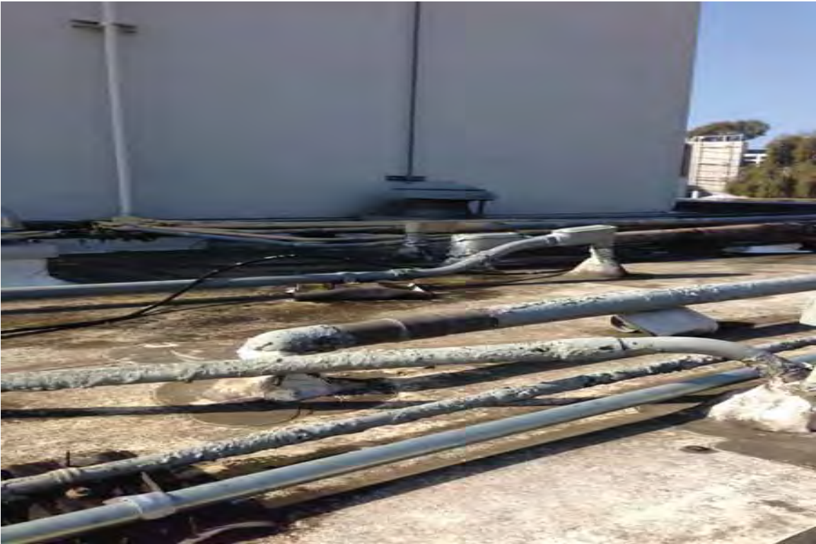
Photographs 17-General view of the suspect roofing materials
