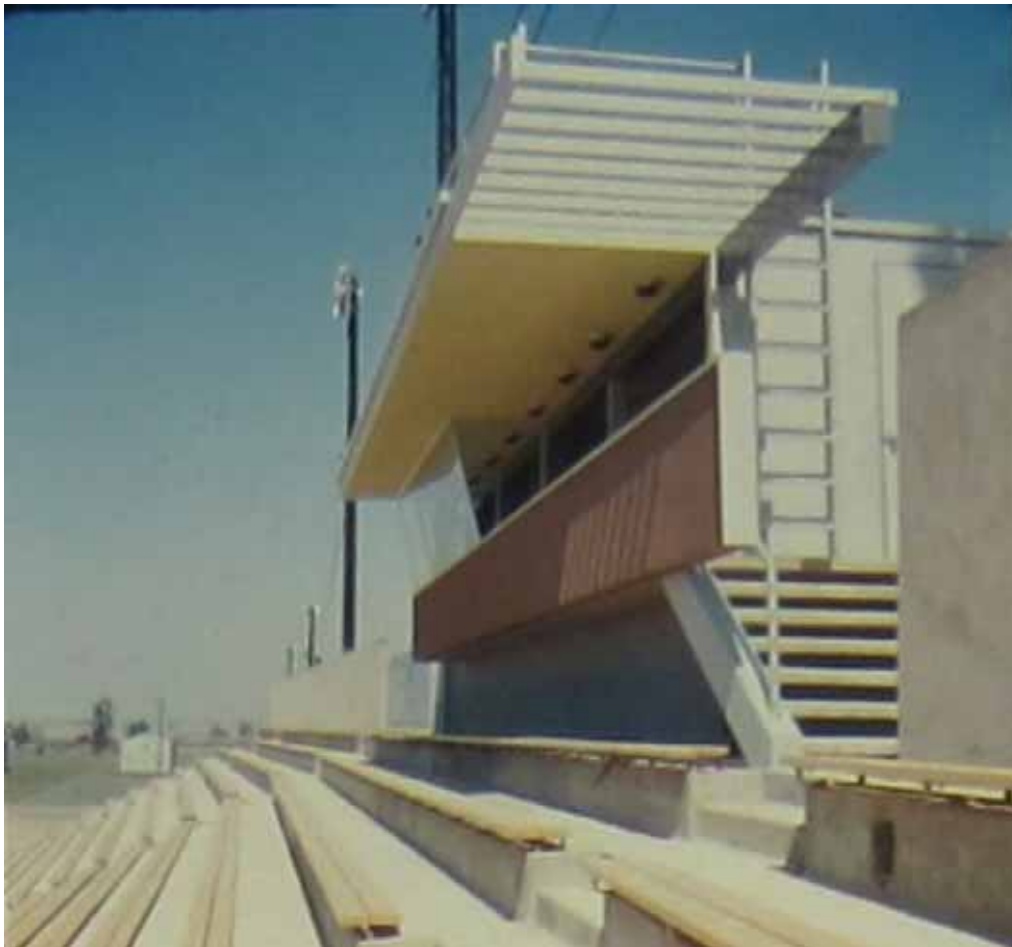
Figure 1D-34: Historic image of the Stadium and Press Box (Bldg. 105). Photo from Robert E. Alexander Collection, Cornell University.
