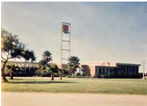
Figure 1B-20: Facing south towards Building 7 (left-hand side) and Building 8 (right-hand side) prior to the first additions. Date unknown, pre-1955. Source: Box 99, Robert Evans Alexander papers, #3087. Division of Rare and Manuscript Collections, Cornell University Library.
