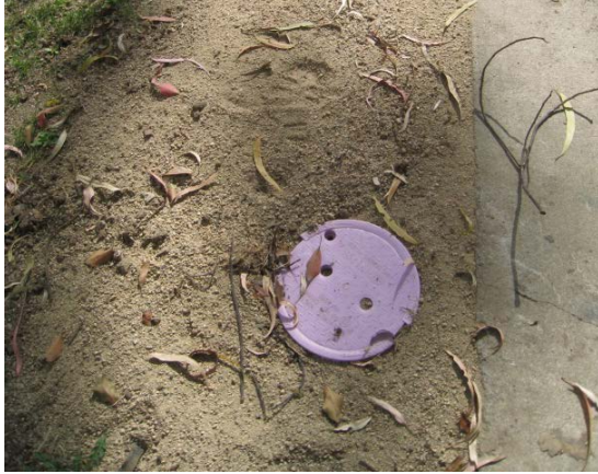
Figure 8. Same location as Figure 5. Map view of water line installation and exposed ground surface.
