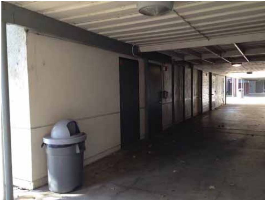
Figure 1C-87: North façade of the Planetarium (Bldg. 39) below the covered walkway.
