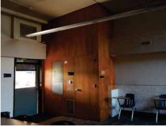
Figure 144: Plywood inbuilt cupboard in Room 104, Building 12.
