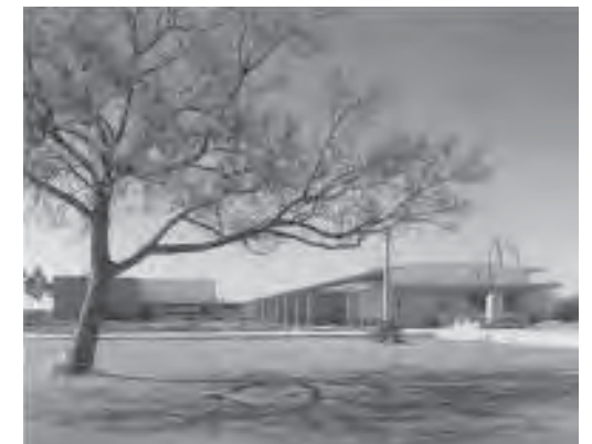
Figure 4: Math and Planetarium complex (Bldgs. 35-37), ca. 1951. Source: Julius Shulman Photography Archive. Copyright The J. Paul Getty Trust. The Getty Research Institute, Los Angeles. ID no.: gri_2004_r_10_b0082_f012_13_2453_01
