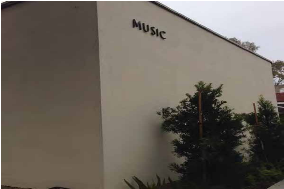
Photograph 11-General view of the suspect exterior building materials
