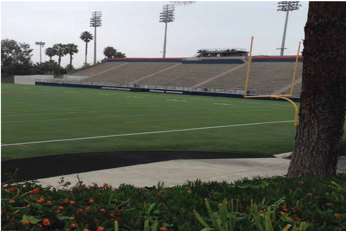
Photograph 9-General view of the Stadium with suspect lead paint
