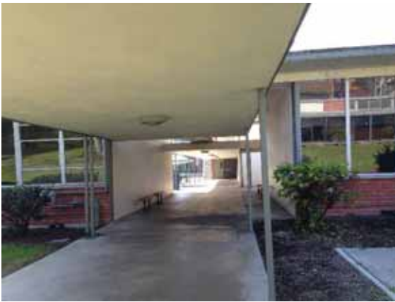
Figure 1C-72: Breezeway between Buildings 35 (left) and 36 (right) towards Building 37. Clerestory windows are present between the walkway canopy and breezeway roof on south façade.
