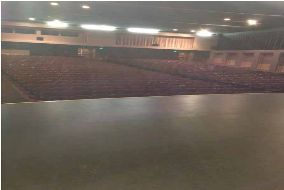
Photograph 4-General view of the interior suspect building materials
