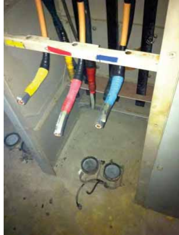
Abandoned 4160V equipment with exposed cables
