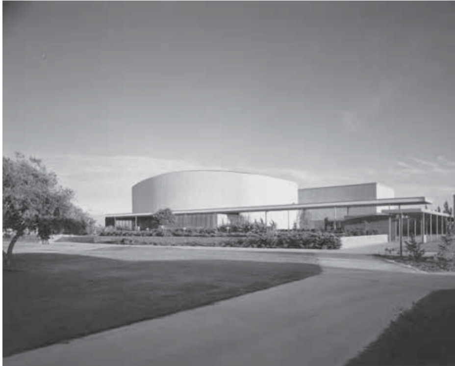
Figure 1B-28: North façade of the Speech Arts Building (Bldg. 2). Date unknown. Julius Shulman Photography Archive. Copyright The J. Paul Getty Trust. The Getty Research Institute, Los Angeles. ID no.: gri_2004_r_10_b0080_f011_1952_51.
