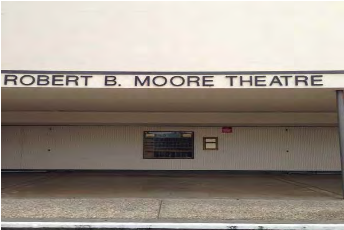
Photograph 1-General view of the building exterior
