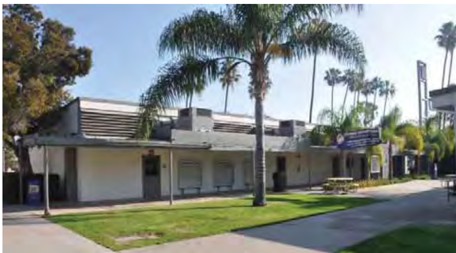
Figure 1C-17: Typical south façade of Building 8 and 9 with louvers covering clerestory windows and added HVAC equipment above the covered walkway.
