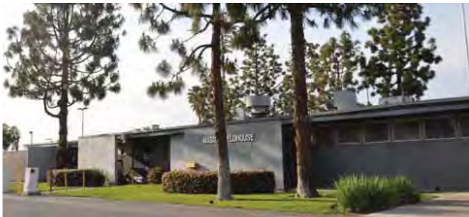
Figure 1C-107: South façade of Feld House (Bldg. 105).
