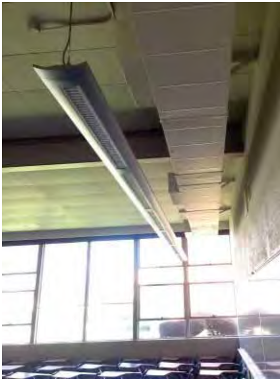
Newly installed lighting
