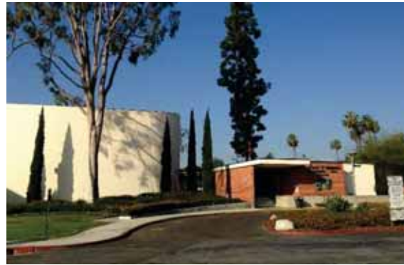
Figure 1C-65: East side of Moore Theater with disabled access ramp and lawn.
