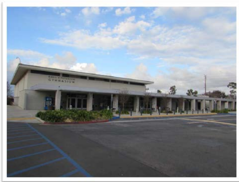
PHOTO - 25: Gymnasium complex, looking north, 2014.
