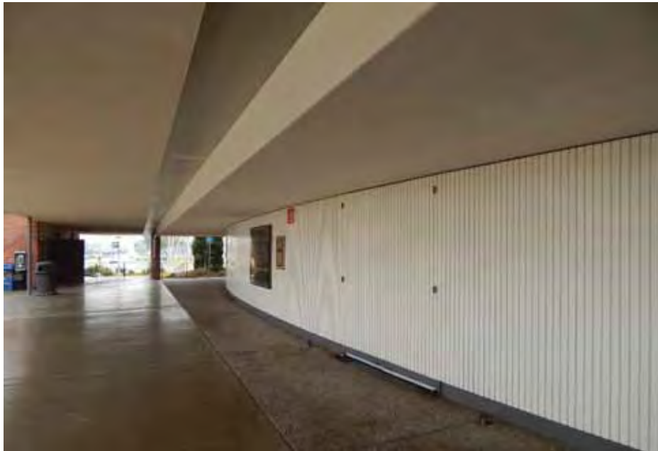
Figure 1C-46: North façade of the Theater, showing the wood siding with hidden doors and soffit above that connects with the covered walkway to create the outdoor lobby. Note the integrated strip of lighting in the covered walkway. Looking east.
