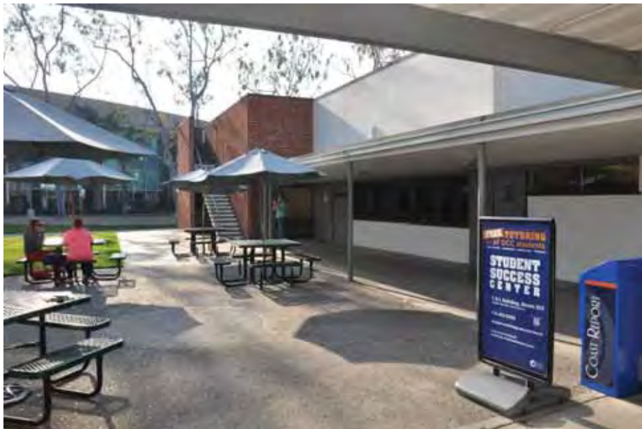
Figure 1B-34: East façade of Building 37.
