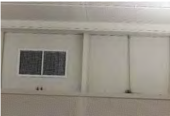
Figure 142: Blocked clerestories in Room 107, Building 13.
