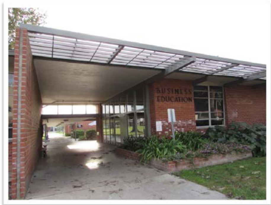
PHOTO - 16: Business Education Building, central corridor, 2014.
