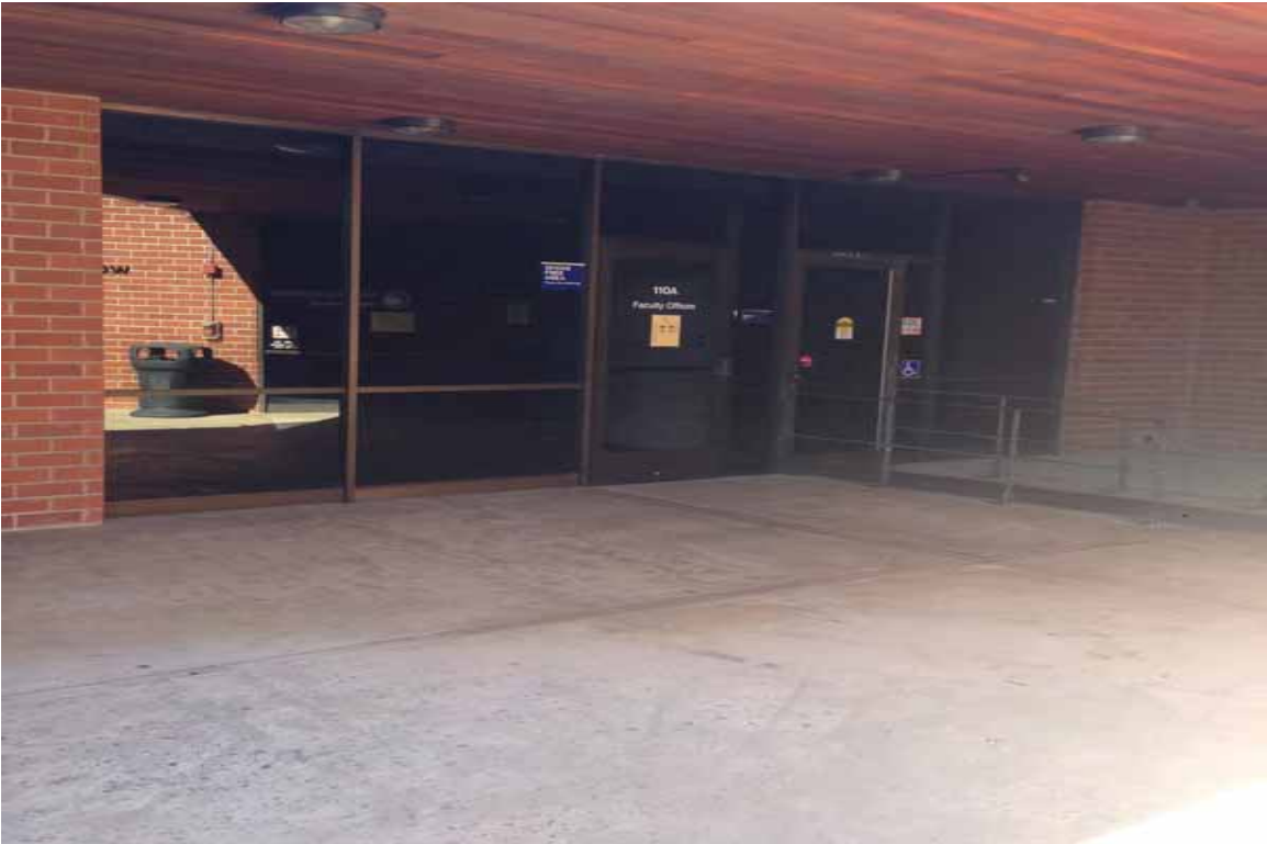
Photograph 5-General view of the exterior building 14
