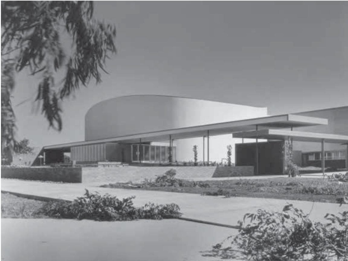
Figure 1D-17: Historic image of the Theater and Music complex (Bldg. 2 & 4). Photo by Julius Shulman, 1955, Getty Research Institute.
