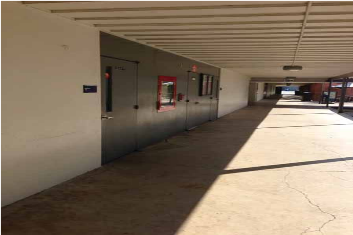
Photograph 1-General front view of the subject buildings 35 & 36
