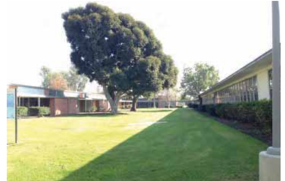
Figure 19: View of quad between Buildings 13 & 36; Building 14 is background center, 2015. Source: Page & Turnbull.
