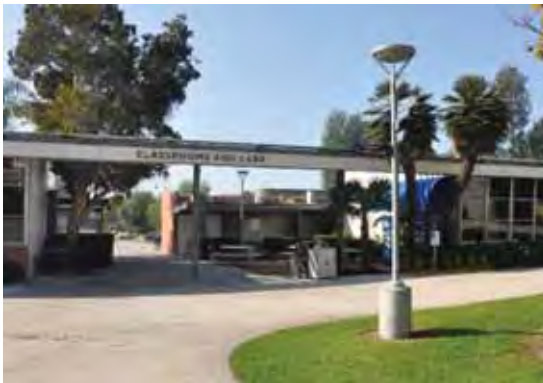
Figure 1C-27: Patio between Bldg. 8 (left) and Bldg. 9 (right) as part of campus circulation, looking southwest.
