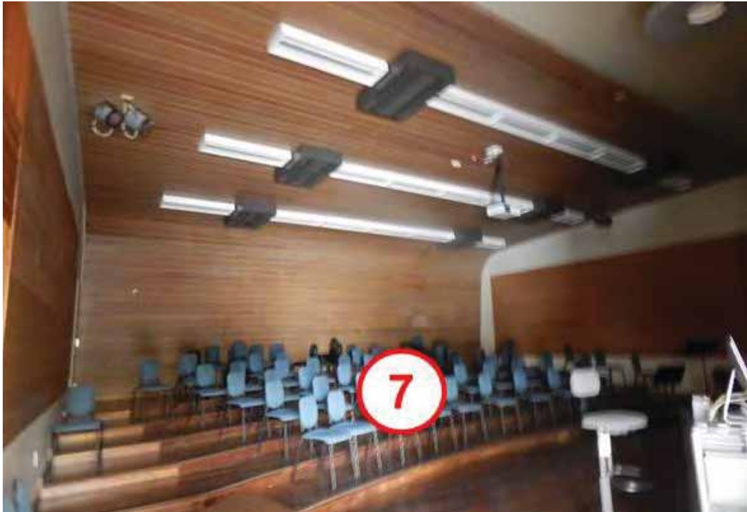
Figure 1D-20: Contemporary image of the Music Building (Bldg. 4) with character defining features identified by red callouts.
