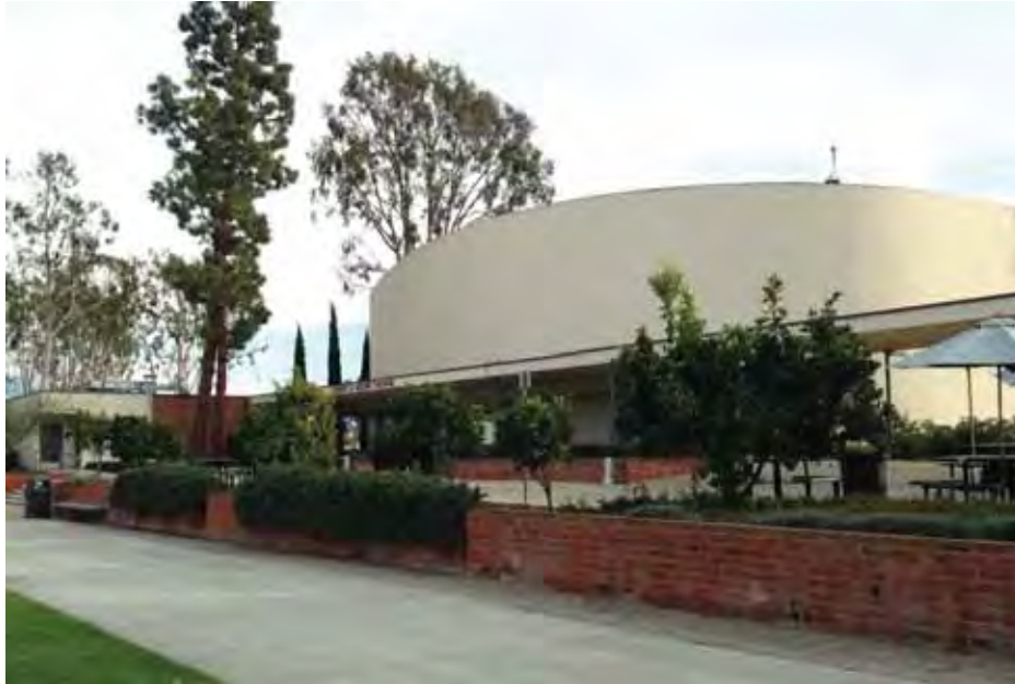
Figure 1C-61: Outdoor lobby at Moore Theater's north side (Bldg. 2). Looking southeast.
