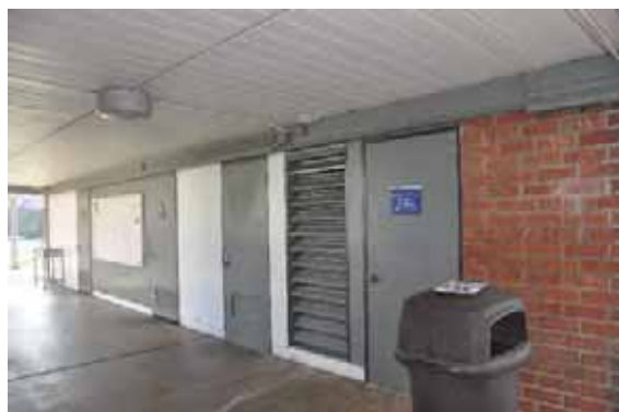
Figure 1C-23: Building 9b's north façade below covered walkway and across from Building 9.
