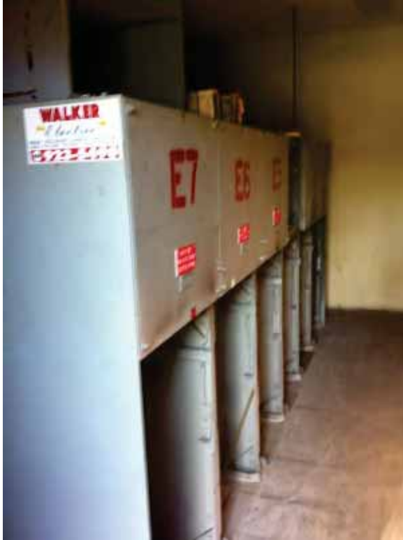
Abandoned 4160V equipment with exposed cables
