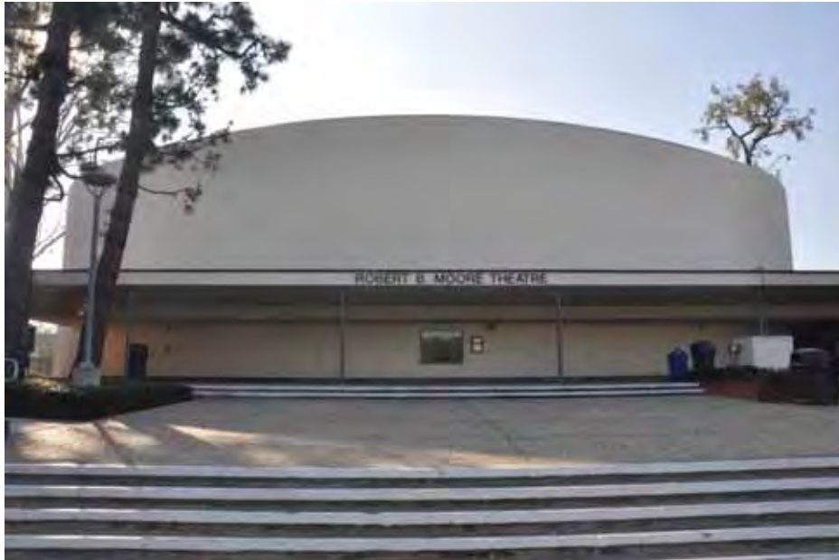
Figure 1C-45: North façade of the Theater, showing the board formed curved concrete wall and tiered landscaping, looking south.
