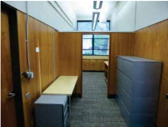
Figure 190: Original plywood paneling and cabinetry in room 150, Building 35.
