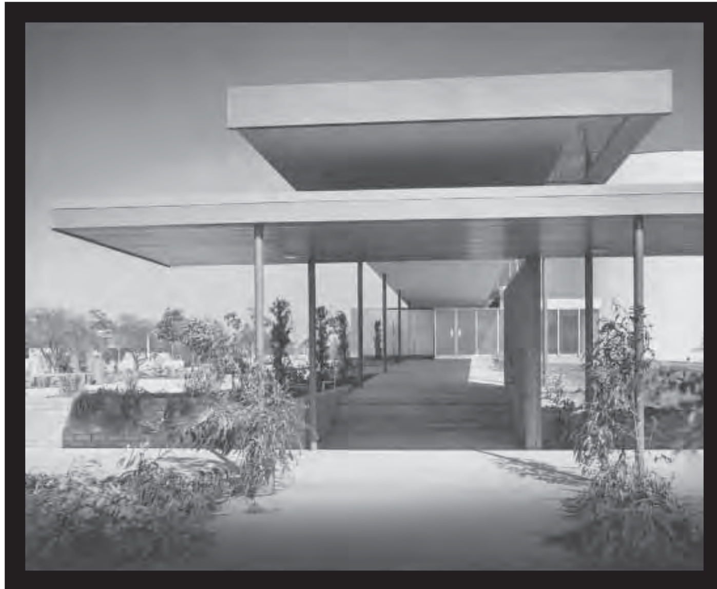
Covered walkway extending from the theater (Robert Moore Theater, Bldg. 2), looking east; ca. 1955. Julius Shulman Photography Archive. Copyright The J. Paul Getty Trust. The Getty Research Institute, Los Angeles.
