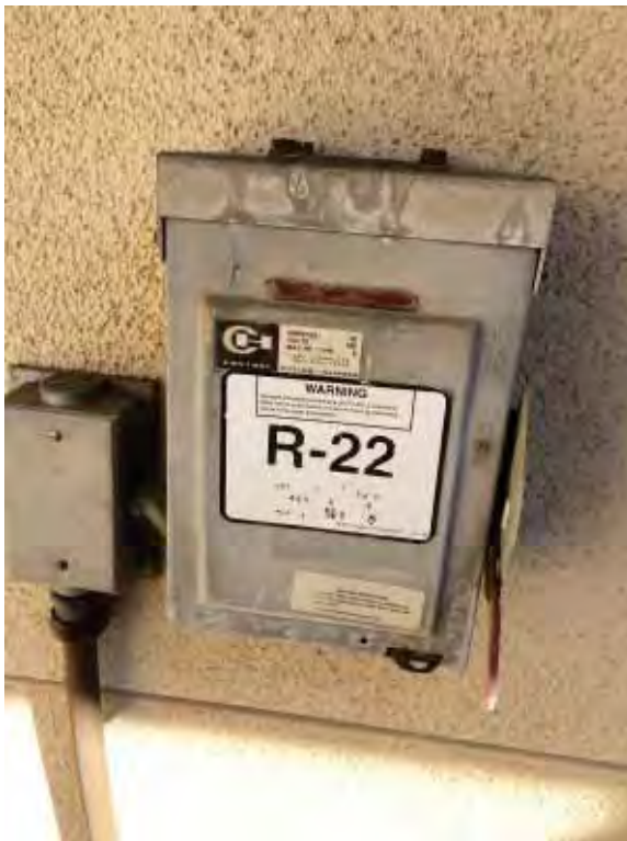
Existing fused disconnect
