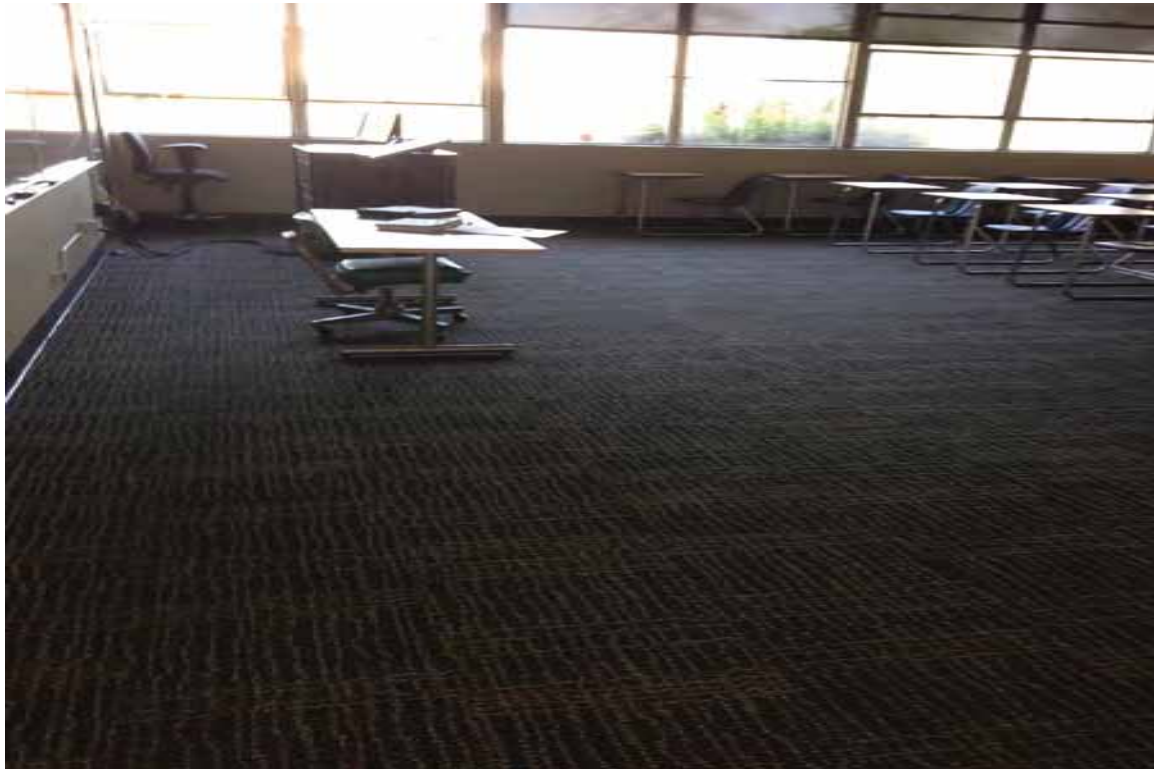
Photograph 4-General view of the interior suspect building materials
