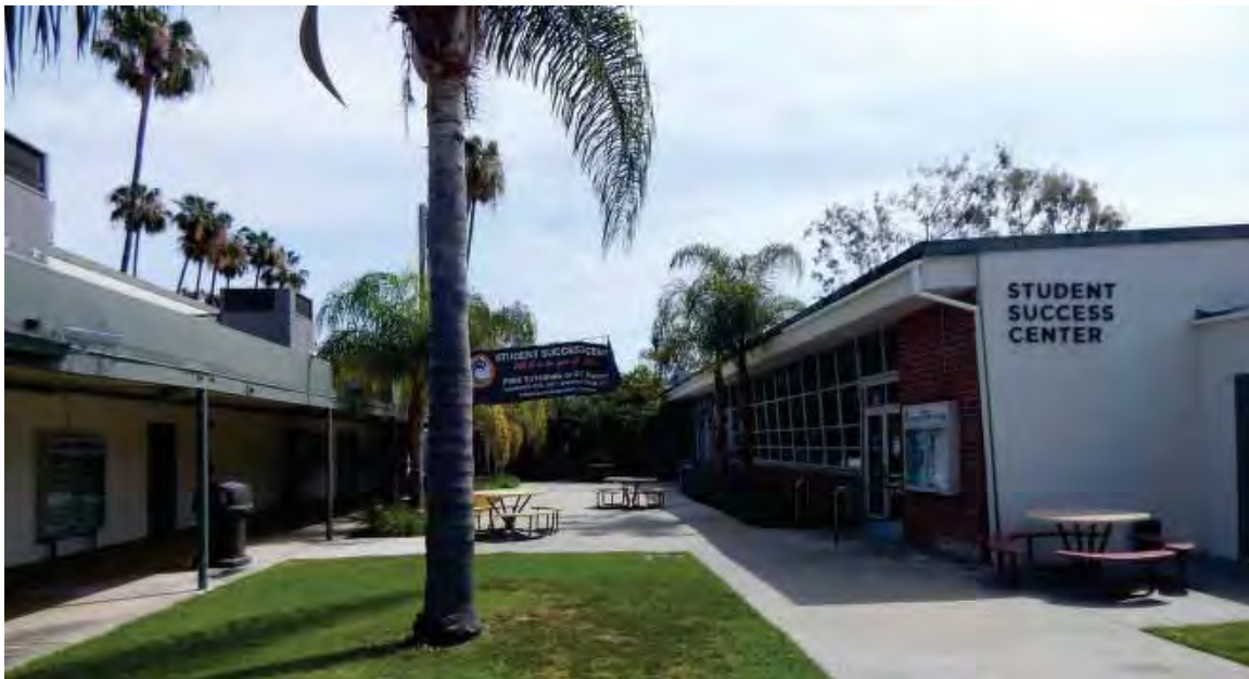
Figure 1 i : The Student Success Center and Classroom & Labs complex (Bldgs. 7-9), facing plan east. ii
