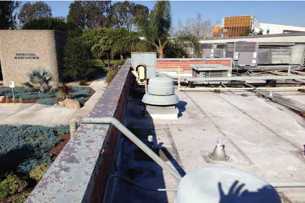
Photograph 12-View of the suspect asbestos and lead-containing roofing materials
