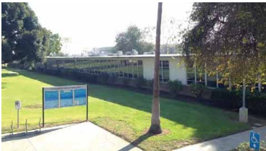
Figure 1C-71: North façade of Building 36 with two stucco panels in the glazed wall marking the later addition.
