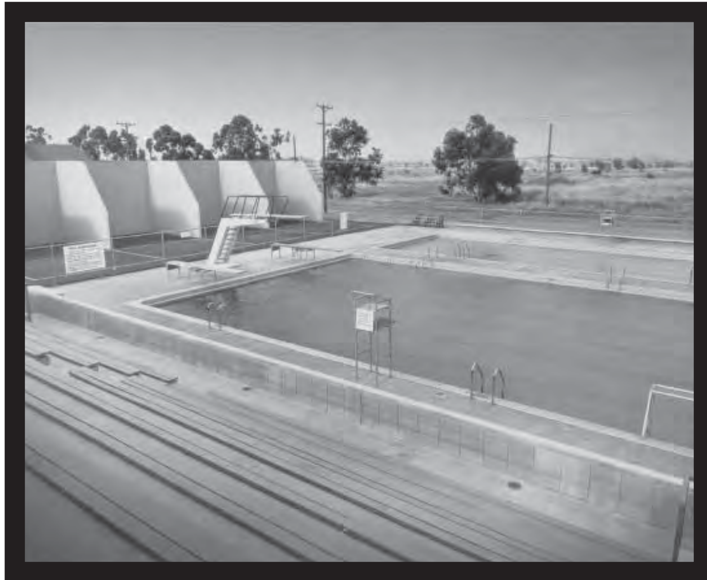
Swimming Pool and Bleachers (Bldg. 93), looking northeast; ca. 1954. Julius Shulman Photography Archive. Copyright The J. Paul Getty Trust. The Getty Research Institute, Los Angeles.
