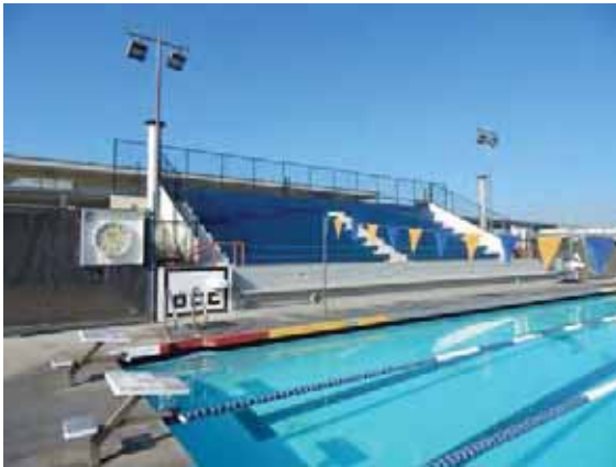
Figure 1C-99: Pool bleachers with CMU wall at its base, looking northwest.
