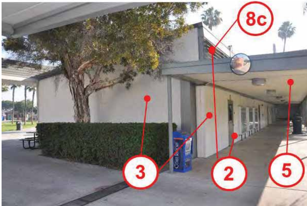
Figure 1D-7: Contemporary image of the Student Success Center and Classroom & Labs complex (Bldg. 8 in photograph) with character defining features identified by red callouts.
