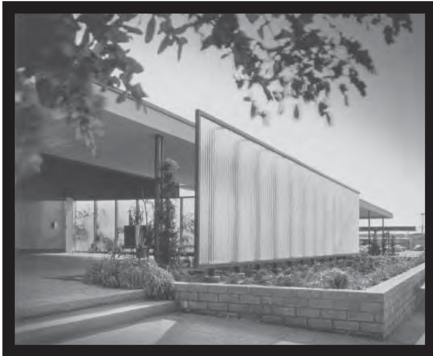
Obscured Glass screening wall along the north elevation of the Theater (Robert Moore Theater, Bldg. 2), looking southwest; ca. 1955. Julius Shulman Photography Archive. Copyright The J. Paul Getty Trust. The Getty Research Institute, Los Angeles.
