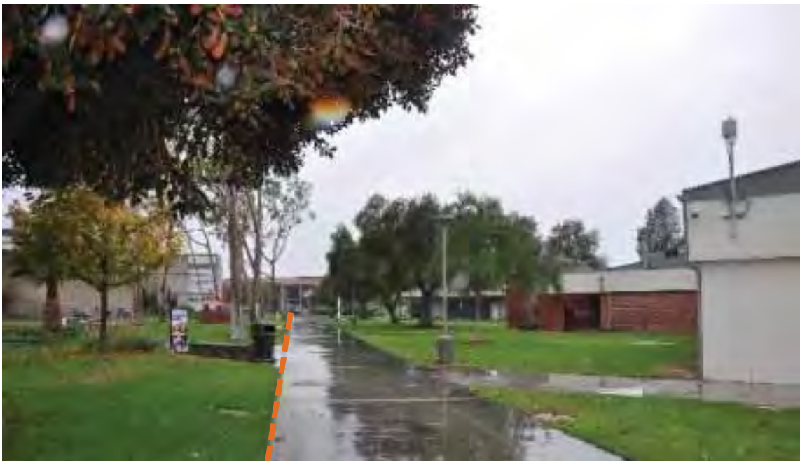
Figure 1C-119: Historic District's south boundary along axial walkway with Historic District to the left (Bldg. 7 in the foreground), looking west toward the Library (Bldg. 182).
