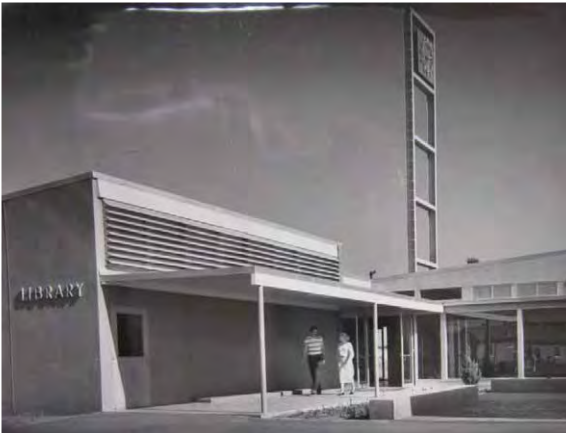
Figure 1D-5: Historic image of the Student Success Center and Classroom & Labs complex (Bldgs. 7 & 8 in image). Photo from Robert E. Alexander Collection, ca. mid-1950s, Cornell University.
