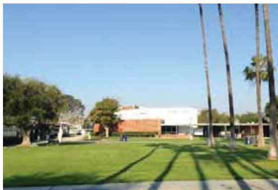
Figure 1C-115: The Forum (Bldg. 81, 1960), northeast of the Historic District, looking west. C&L (Bldg. 9) in the Historic District is to the left.
