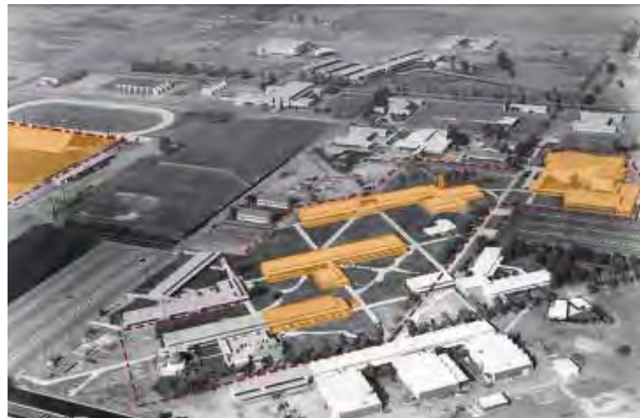
Figure AX: 1959 Aerial of Orange Coast College. Buildings highlighted shall be retained as part of Preservation Alternative 1. Source: Orange Coast College Library.
