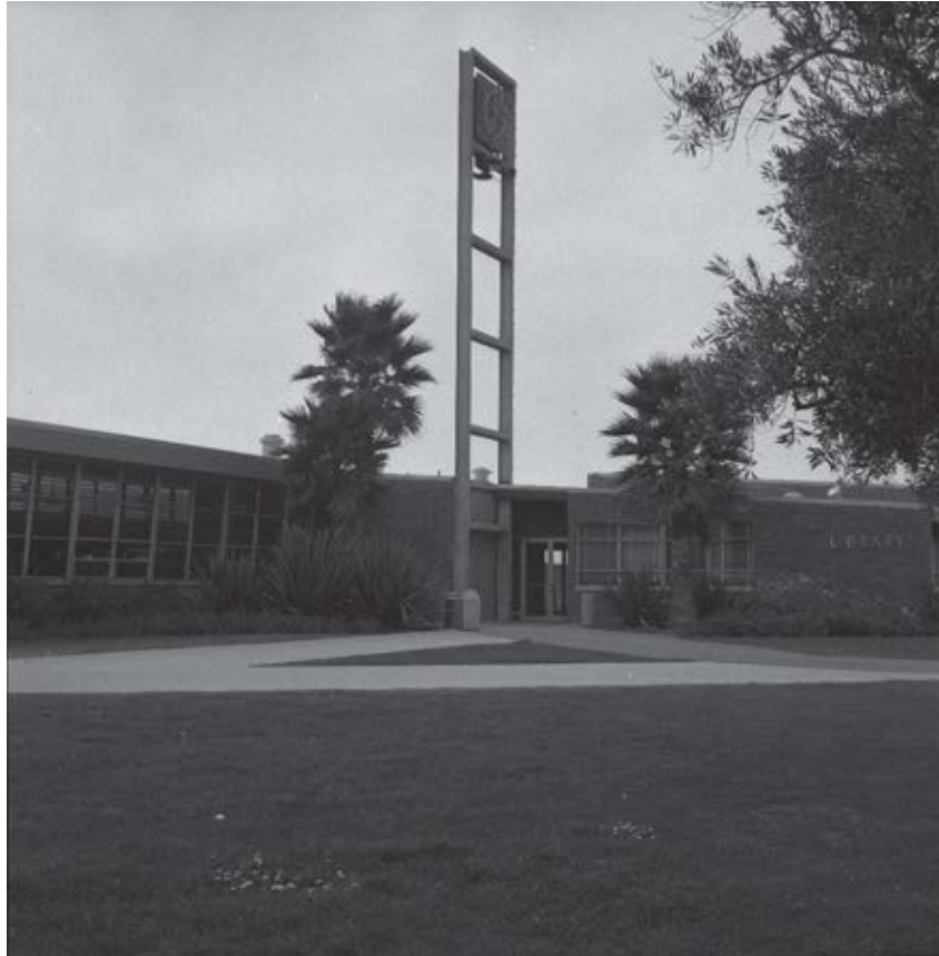
Figure 1B-17: Facing west towards Building 7 (left-hand side) and Building 8 (right-hand side). Glazed doors in position at the east entrance to the walkway between the two buildings. Date unknown. Source: Manu. Box 74 folder 621-622, Garrett Eckbo Collection, Environmental Design Archives, University of California, Berkeley.
