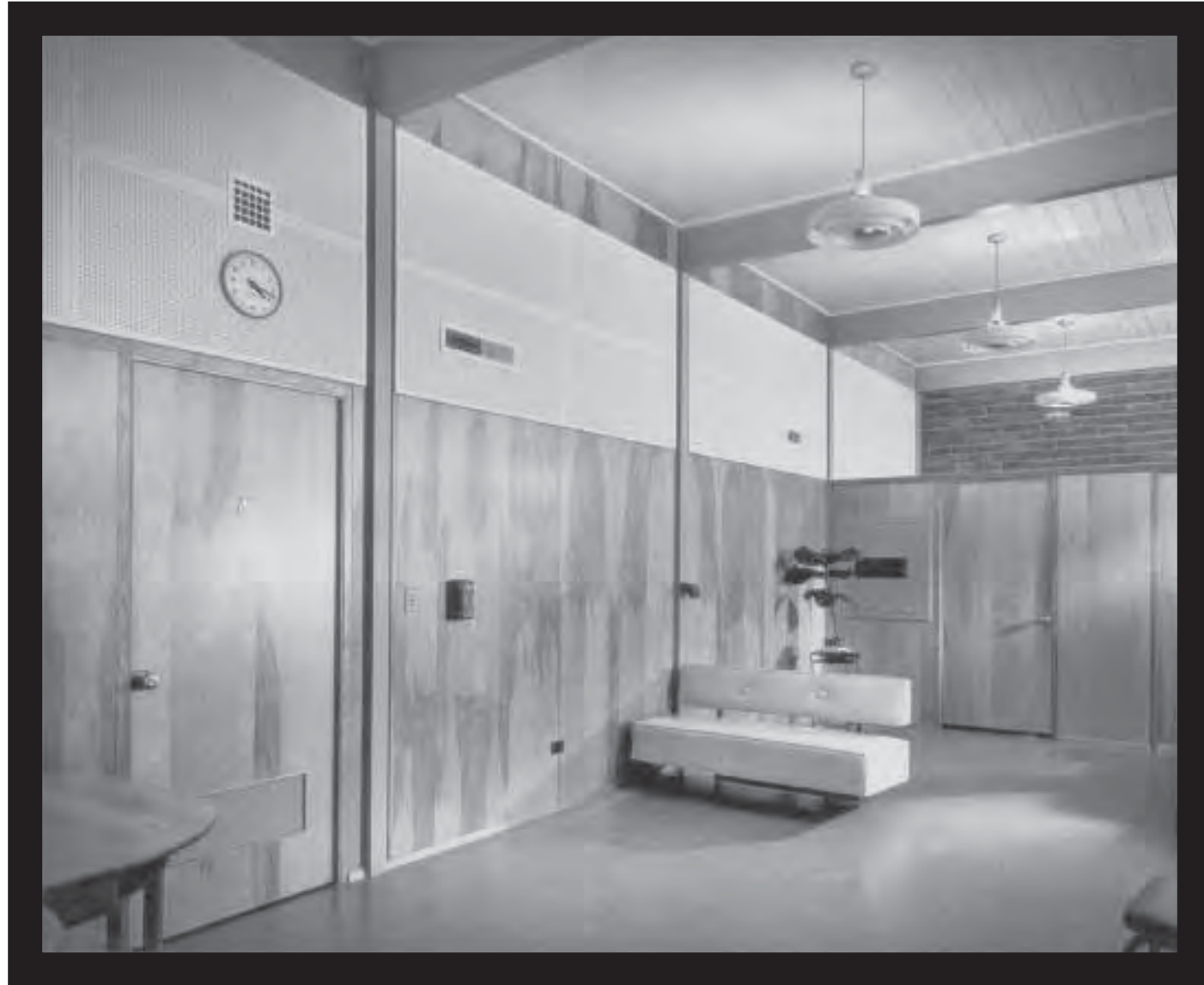
Interior of Business Education Classroom (Business Education, Bldg. 12/13); ca. 1954. Julius Shulman Photography Archive. Copyright The J. Paul Getty Trust. The Getty Research Institute, Los Angeles.
