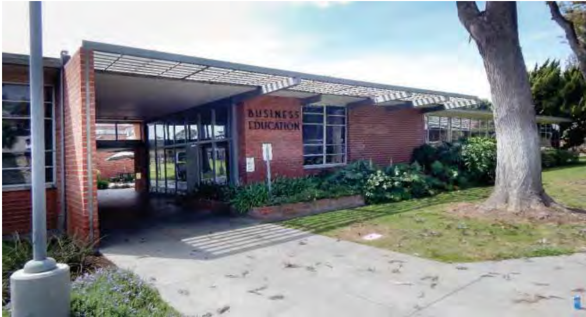
Figure 126: North façade of Business Education west wing (Bldg. 13).
