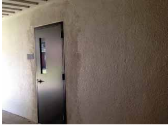
Figure 168: Stucco patching around doorway on Building 36.
