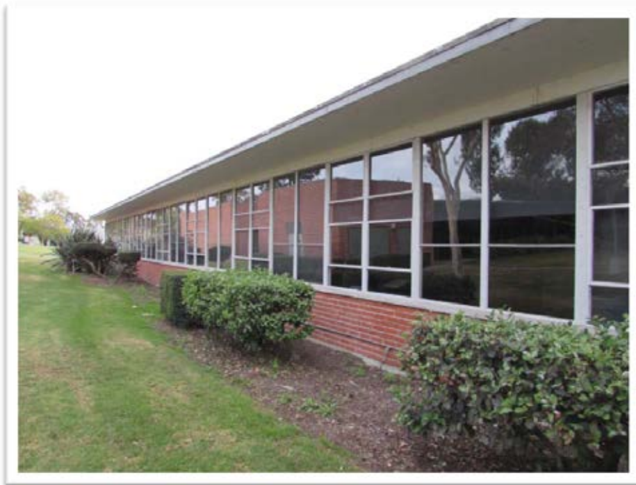
PHOTO - 37: Classroom wing fenestration and canopy overhang details, 2014.
