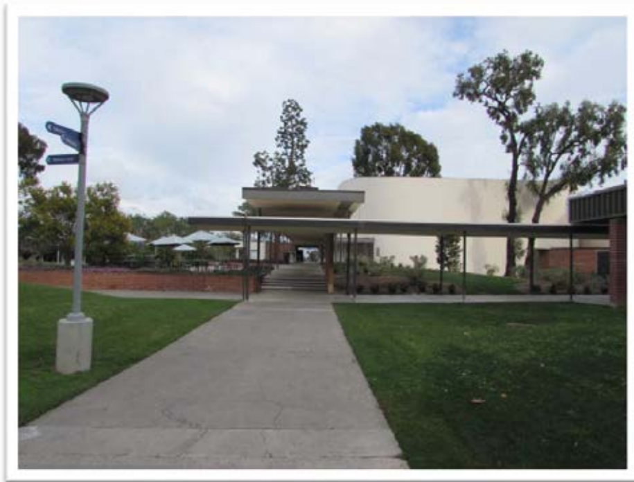
PHOTO - 10: Speech Arts Theatre Building, side view, looking east, 2014.
