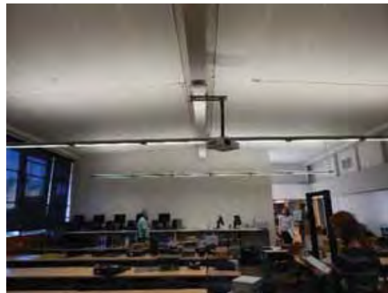
Figure 1B-26: Classroom 106, Building 13. The clerestory windows have been painted or covered, original lighting fixtures replaced and the internal wall partition has been altered.
